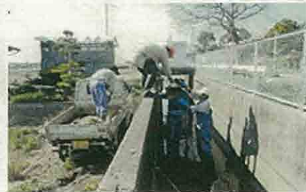
Dredging earth and sand from waterways
