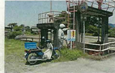
Patrol and checkout of irrigation channels
