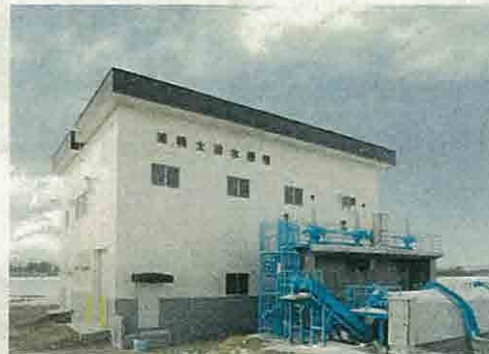
Drainage pump station
