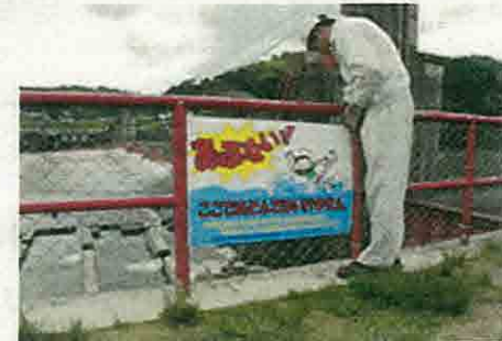
Installing warning signs
