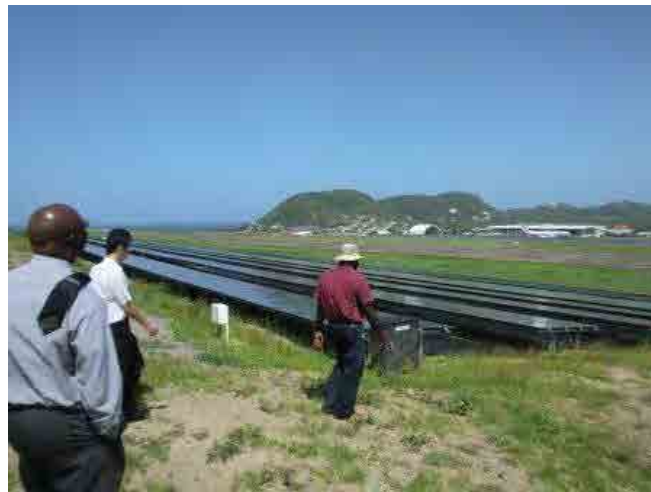
Figure 4 750kW Solar farm (St. Christopher and Nevis)
