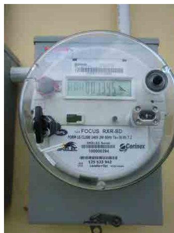
Figure 10 Smart Meter (St. Christopher and Nevis: Landis+Gyr Production)
