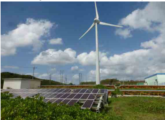
4 November, 2014 Exterior of Mega-Solar Facilities and Wind Turbine in Miyako Island
