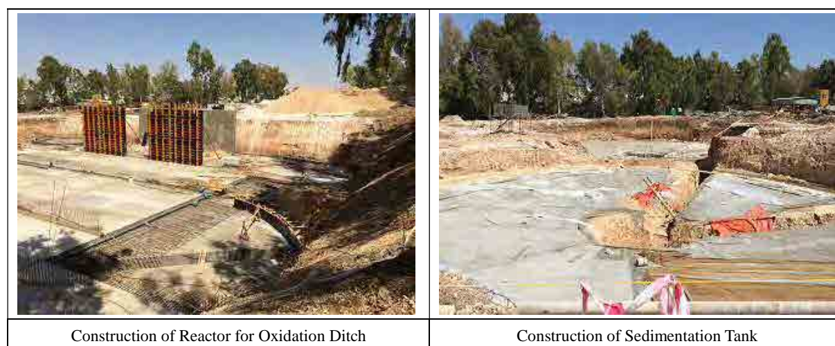
Figure 3.11 Rehabilitation Financed by KfW at Central Irbid WWTP
