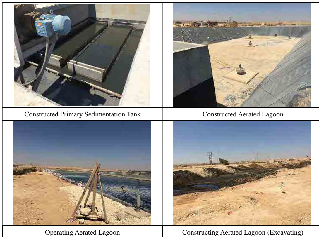
Figure 3.10 Upgraded and Constructing Facilities at Mafraq WWTP
