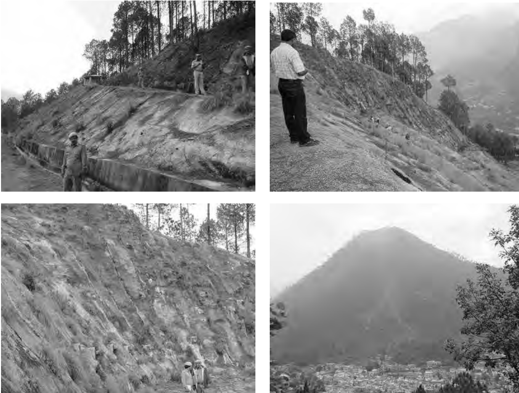
Observation of slope failure stabilization work on Mt. Varunawat
