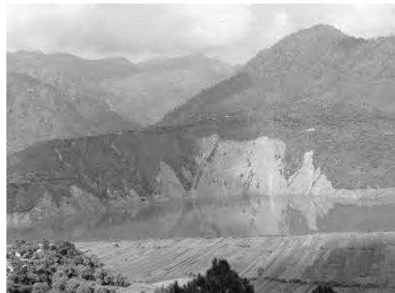
Slope failure along the backwater of Tehli Dam
