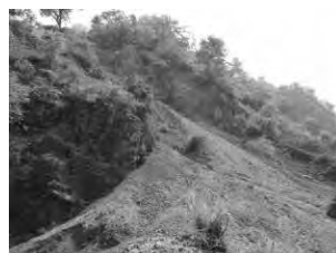
Top of the landslide
