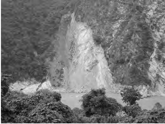
Slope failure at Nar Kota Village. A small foot pass is collapsed by slope failure.
