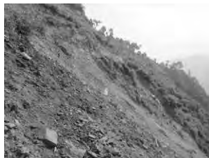
Top part of slope failure
