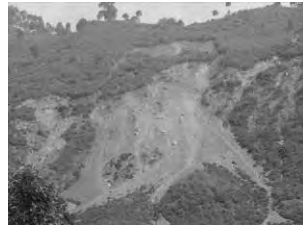
Full view of slope failure - 2
