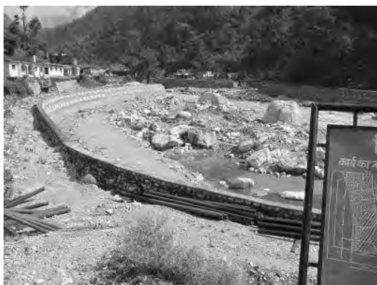
Flood protection works at the Assi Ganga River
