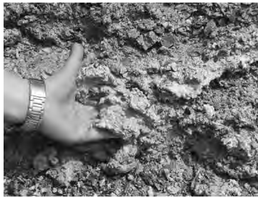
Clay soil, the cause of landslide
