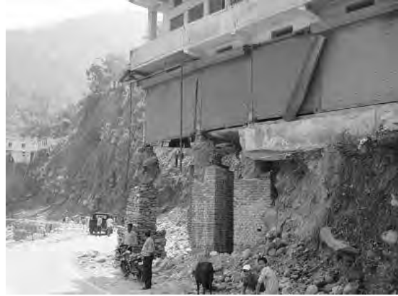
Damage situation by river water flow at Vijaynagar Village
