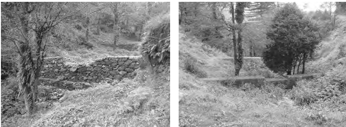
Civil works along the Magra River by UKFD
