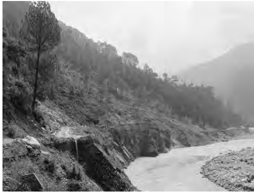
Landslide site along the Bhagirathi River
