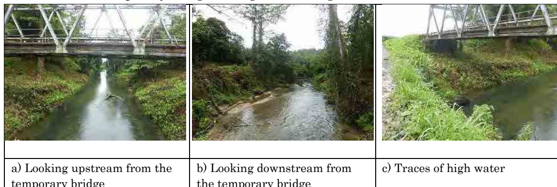
Figure 2.2.5 River Channel Conditions around Aum Bridge
