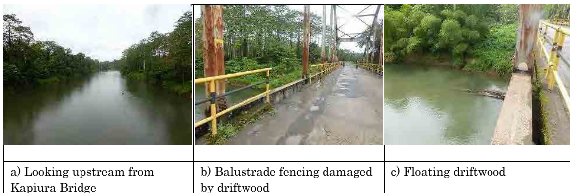
Figure 2.2.4 River Channel Conditions around Kapiura Bridge
