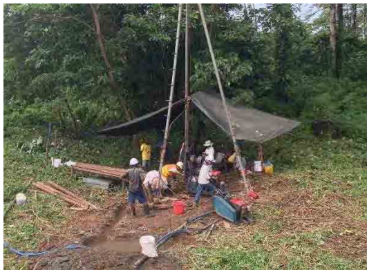
Photograph 1.2.1 Kapiura Left Bank Boring
