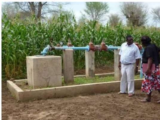
Groundwater Borehole with Submersible Motor Pump
