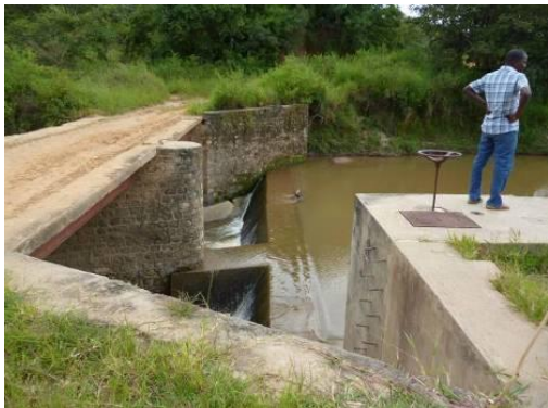
Problem with Sand Sedimentation around the Intake in Mzimba
