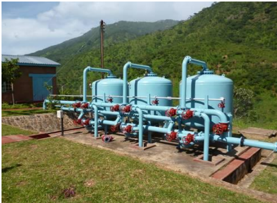
Pressure Tank Filtration
