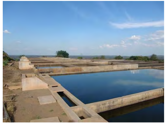
Water Treatment Plant in Zomba
