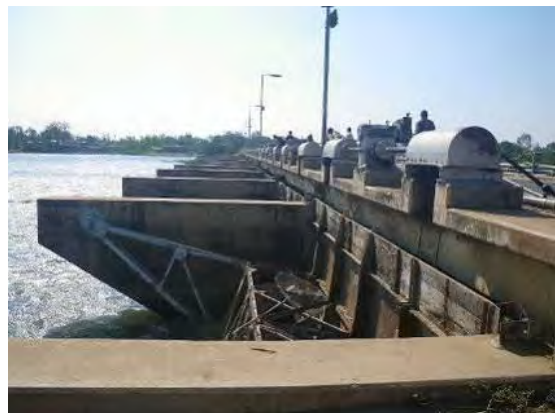
Kamuzu Barrage at Liwonde
