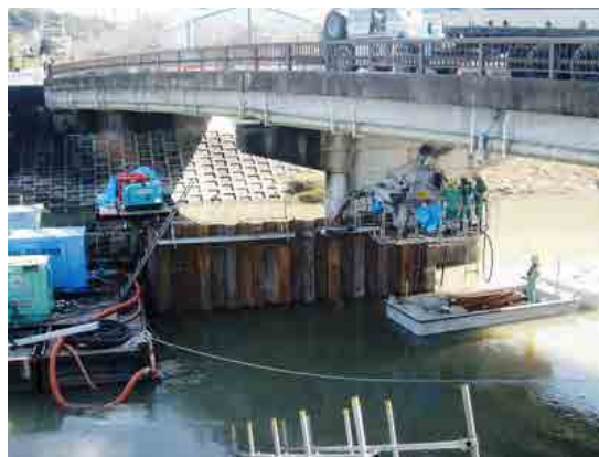
Figure 2-2-34 Sample of Steel Sheet Piling under Bridge
