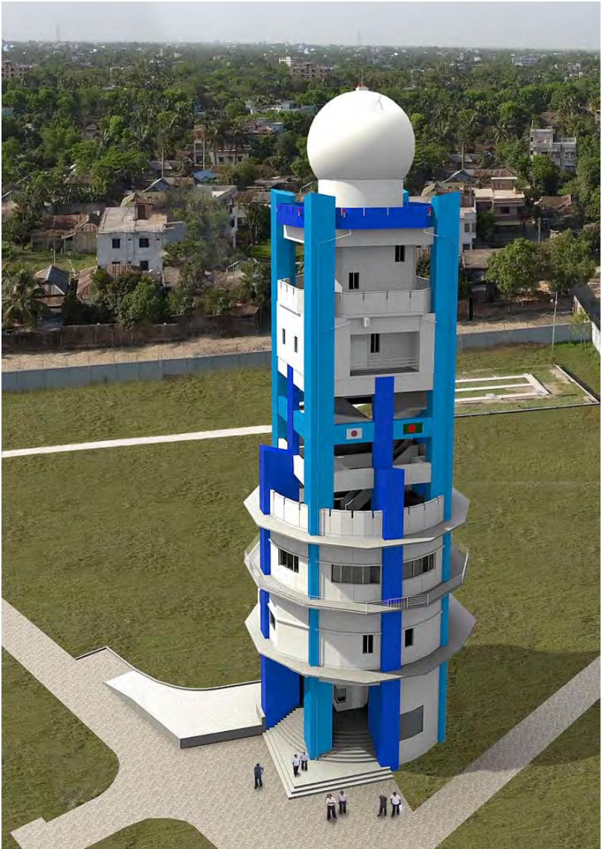
Rangpur Meteorological Radar Tower Building
