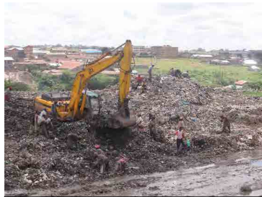
Waste picking activity during spreading of waste by excavator
