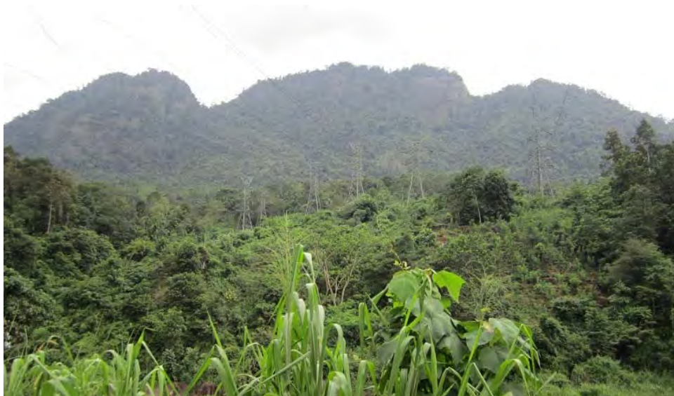
Existing T/L in front of GS
