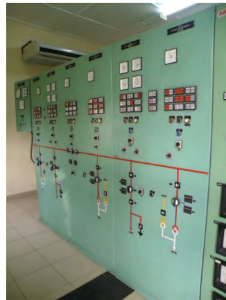
Existing 132kV Protection & control facility to be replaced
