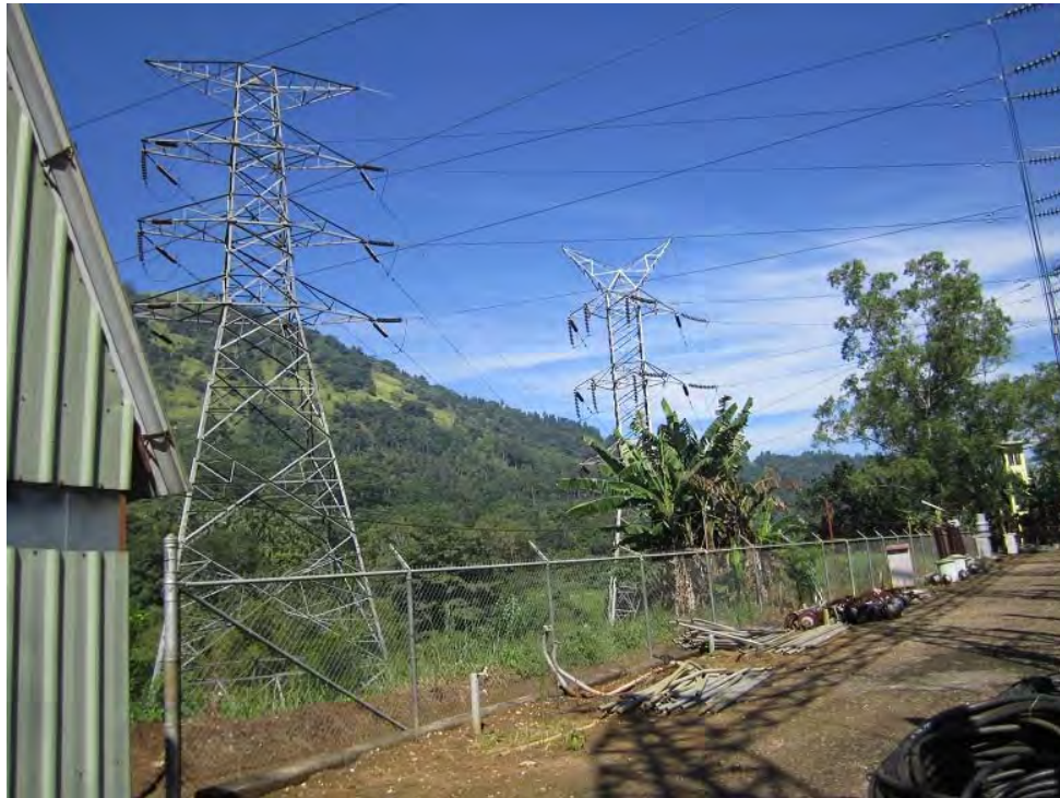
Existing 132kV Kiribathkumbura / Habarana dead-end tower (Remove existing tower and construct new tower)
