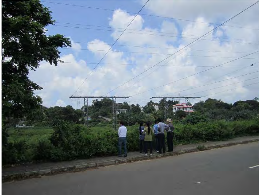
Existing 132kV Kolonnawa – Aturugiriya lines go under 220kV T/L
