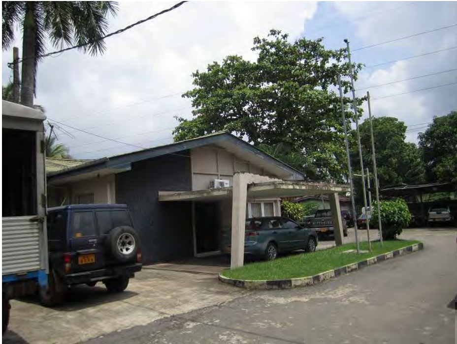
Figure 6-2 Office of D.G.M (O&M) Building
