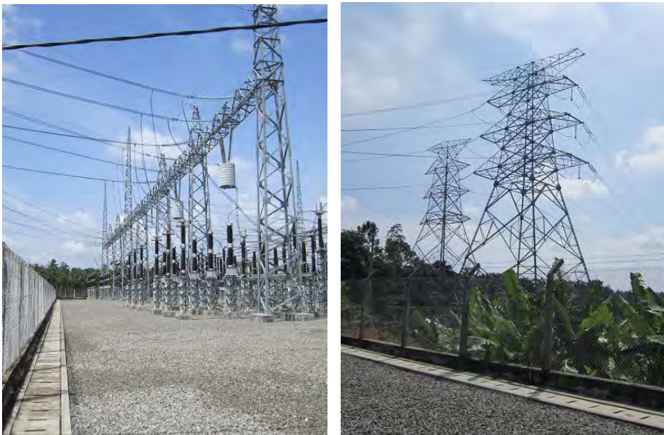
Same scale gantries and tower (Double Zebra) will be constructed.
