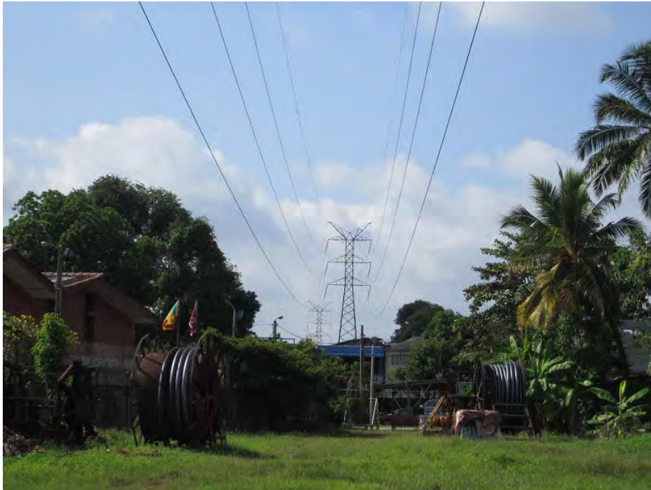
Existing 132kV Kolonnawa– Pannipitiya line (No2 and No3 tower are seen )
