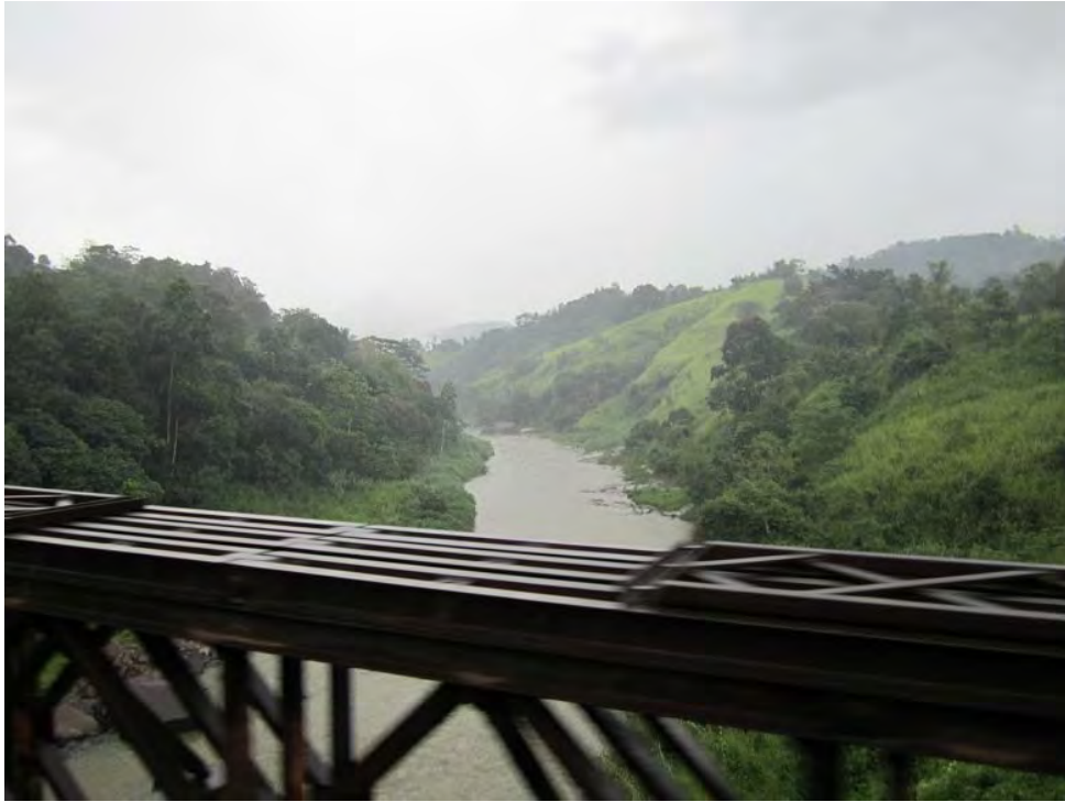
New T/L goes along with the river here (Near Ulapane town)
