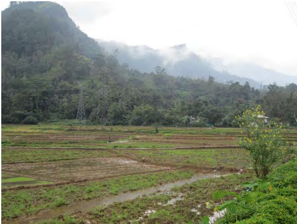
New T/L goes along with existing 132kV line here
