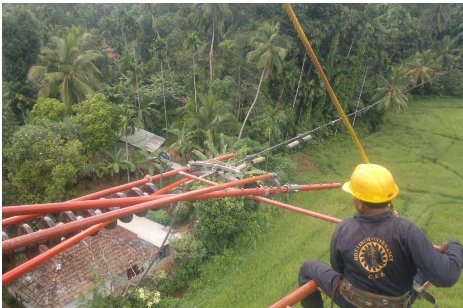
Figure 6-4 Stick Tool for hot line (When they change insulator, they connect attachment to stick tool like this)
