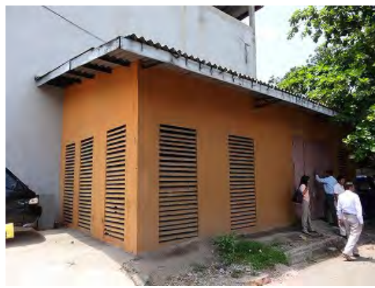
RSS building (CEB Colombo City Area) Size: (D)5 m × (W)10m (7m in case of without Tr)
