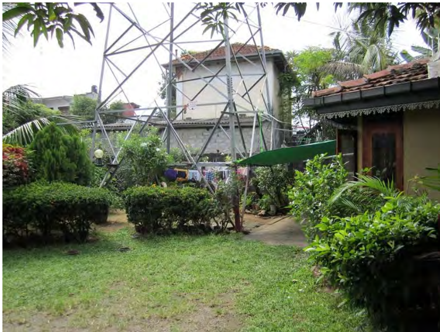
Existing 132kV Kolonnawa No.4 tower (The tower is located inside a private garden.)
