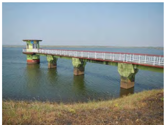
Figure 6-3-12 Intake Tower at Aline Nee
