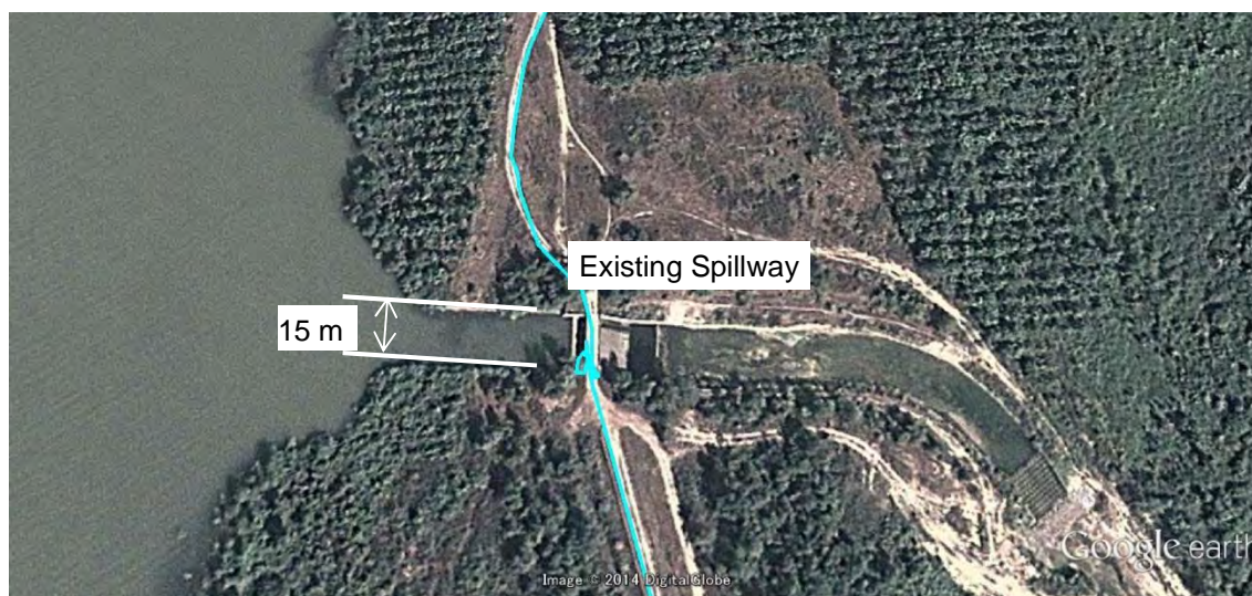
Figure 6-3-14 Location of Spillway at La Gun Byin Reservoir
