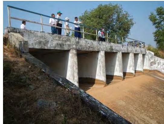
Figure 6-3-8 Spillway Bridge at La Gun Byin
