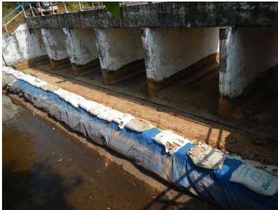
Figure 6-3-7 Spillway Crest at La Gun Byin
