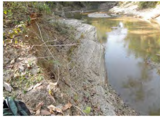
Figure 6-4-8 Left Abutment at Dam Site
