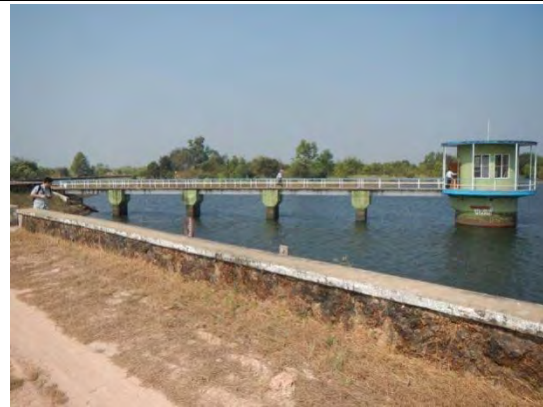
Figure 6-3-6 Intake Tower at La Gun Byin
