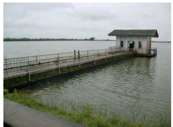
Figure 6-1-5 Intake Facility (Pumping Station)
