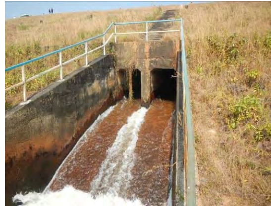
Figure 6-3-10 Outlet Work at La Gun Byin
