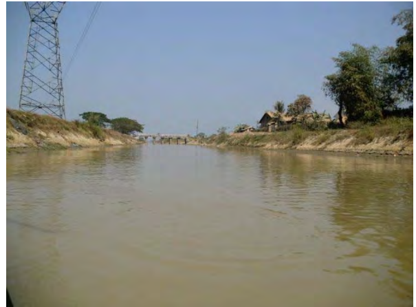
Figure 6-2-26 Main Canal of 30 Miles Greening Project
