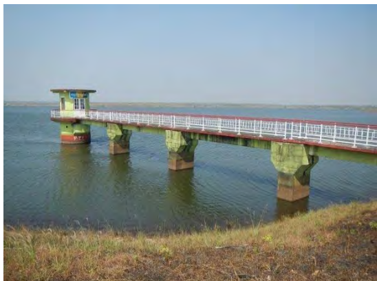
Ailne Nee reservoir and intake facility (January 2014)
