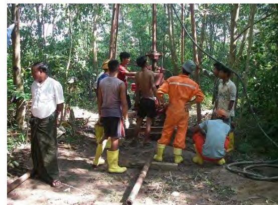
Borehole drilling (D-2 site) (February 2013)
