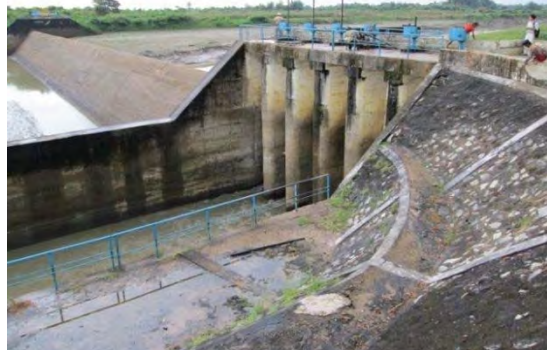
Zaung Tu weir (February 2012)
