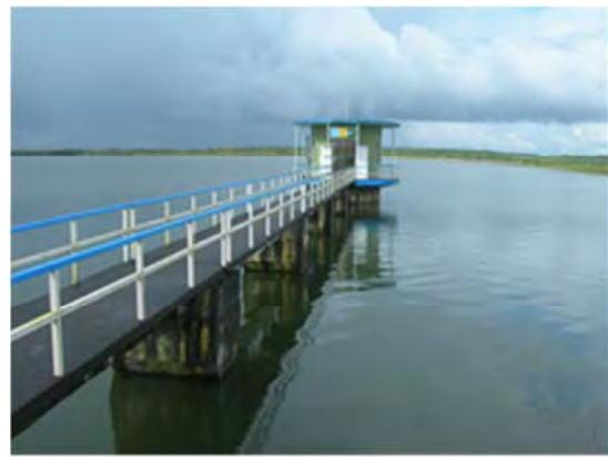
La Gun Byin reservoir and intake facility (November 2012)
