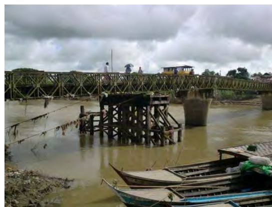
Existing river water level gauging station at Bago river (October 2012)
