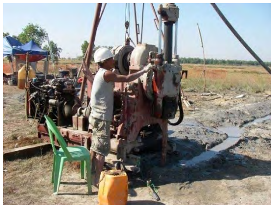
Test well drilling (D-1 site) (December 2012)
