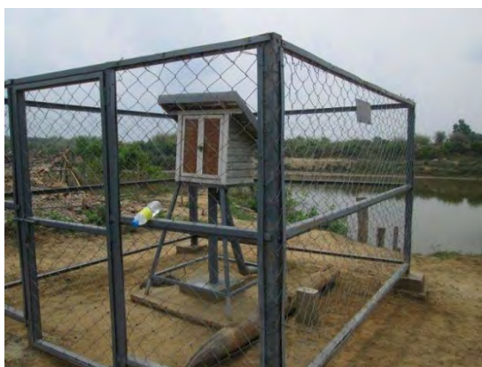
Automatic river water level gauging station at Tamabin (May 2014)
