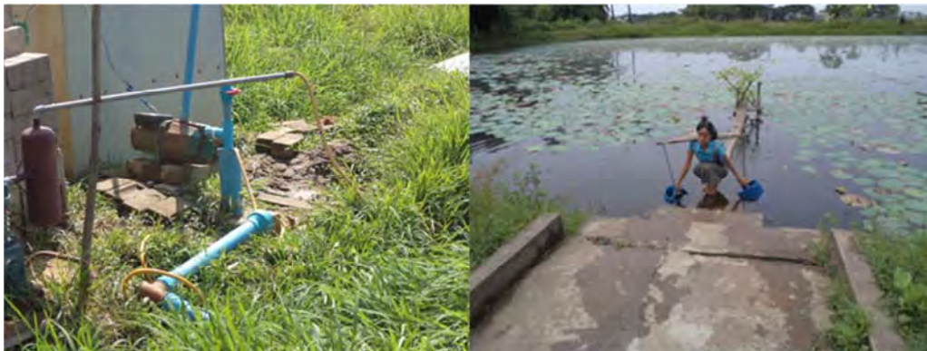
Tube well with airlift pump (Thanlyin)
