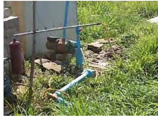
Existing deep well in Thanlyin township (November 2012)
