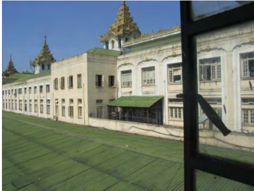
Pic-13: We look new signal cabin from existing signal cabin. There are 3 rd floor in the main building.
