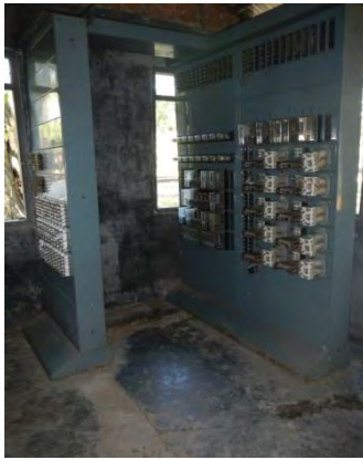
Pic-39 TMS station device is installed in signal equipment room of each station. Information is obtained also from existing equipment in part (Panugdawthi station)
