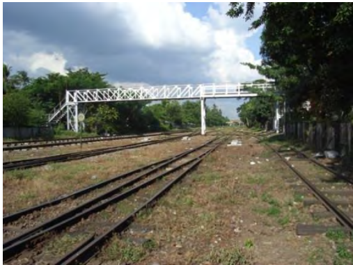
Pic-15: The Pazundaung station yard 1.6km away from Yangon central Station. The loop line and the main line are grade crossing.
