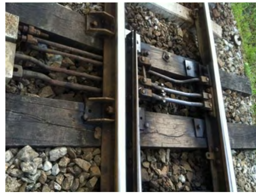
Pic-20: Parts of Equipment of interlocking . It is connected by different method unlike Japanese general specifications.
