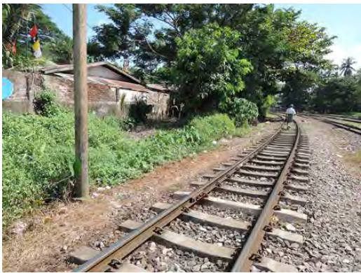
Pic-27: A low voltage electrical power cable at Pazundaung Station from the north side of Yangon central station will be buried.
