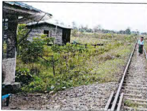
SW1: Warning device for level crossing SW2: Control for barrier machine
