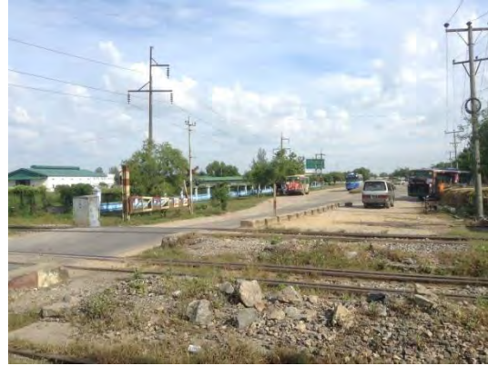
Pic-32: The schedule to which maintenance of ballast is also performed simultaneously with formation of an automatic alarm.
