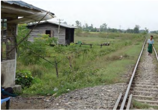
Pic-37: Installation schedule place of automated level crossing control device and diesel generator. A retaining wall is needed.
