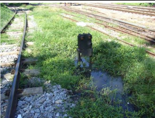
Pic-11: In South-East side of Yangon central station, domestic wastewater is directed to the station and submerges signals.
