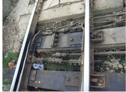
Pic-8: Parts of Equipment of interlocking. Spare is nothing. It has been used since 1950, while repairing it. The state is not good.
