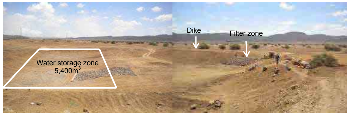
Improvement Work of Kourtimalei Pond (June 2012)
