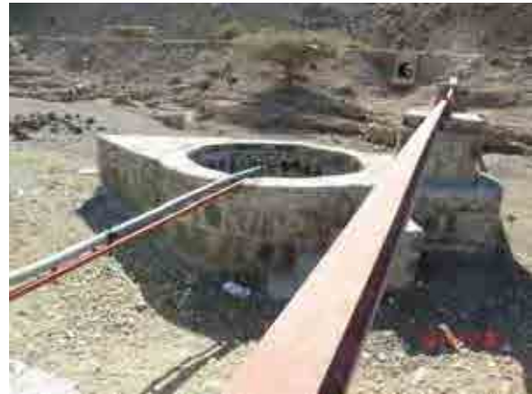
Protection Works of the Shallow Well (Hambokto)
