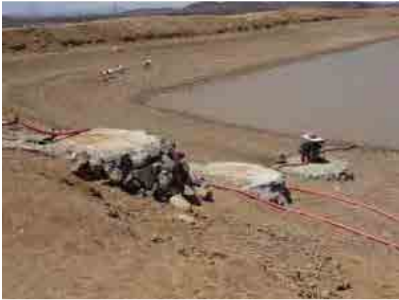
Intake Works (Kourtimalei)
