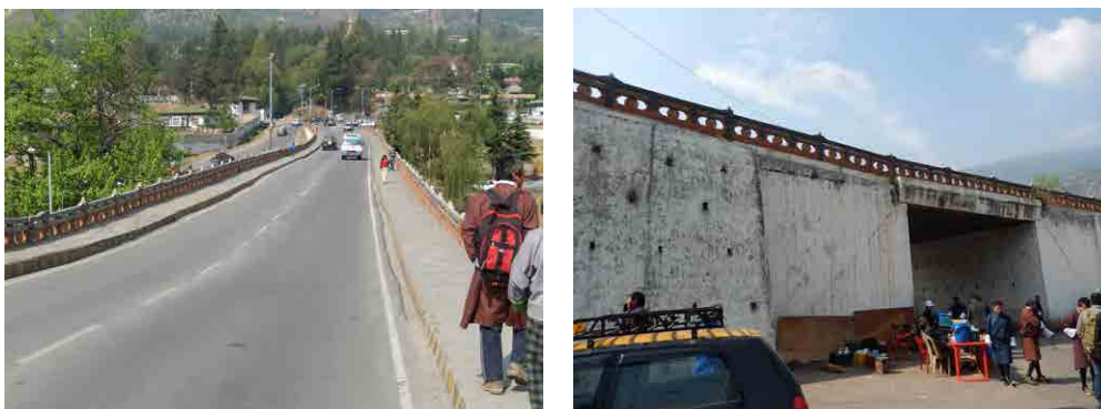
Source: JICA Study Team <Figure8-2> Lungten zam Bridge in Thimphu
