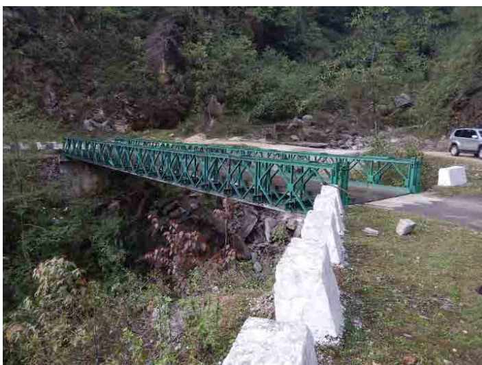
Photo-6 Bridge site survey 2014/4/15~20 A-3.Namling zam Bridge
