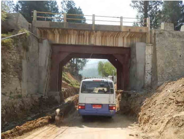
Photo-4 Bridge site survey 2014/4/15~20 A-1.Semtokha Flyover Bridge
