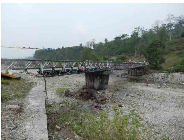
Photo-24 Bridge site survey 2014/4/28~30 C-3.Jitti zam Bridge
