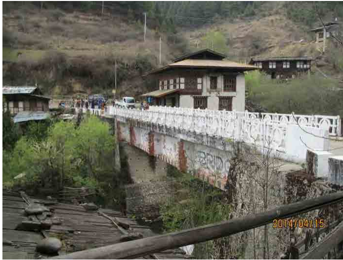
Photo-13 Bridge site survey 2014/4/15~20 A-10.Nikachu zam Bridge
