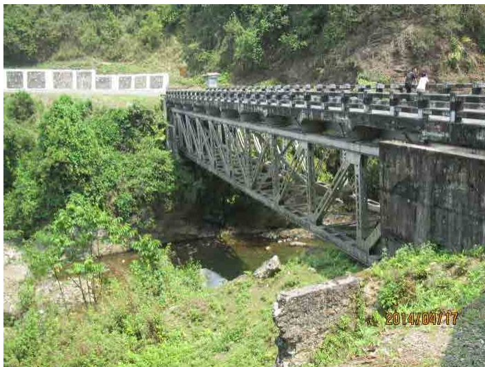
Photo-20 Bridge site survey 2014/4/15~20 B-6.Samkhara zam Bridge
