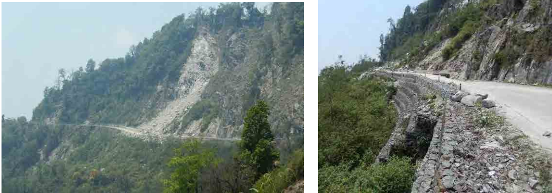
Source: Photos taken by JICA Study Team <Figure4-2> Jumbja landslide
