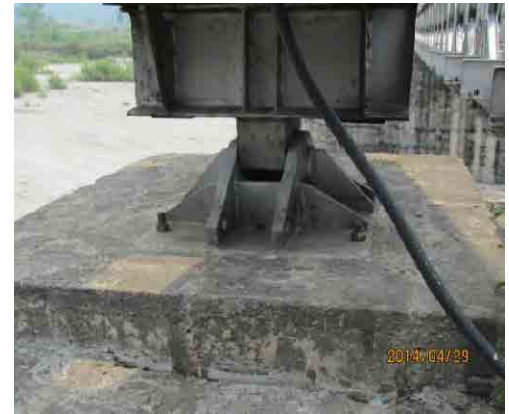
<Figure5-17> Connection status of main tower and the bridge pier and beam
