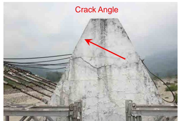
Source: JICA Study Team <Figure5-16> Cracks in the anchorage
