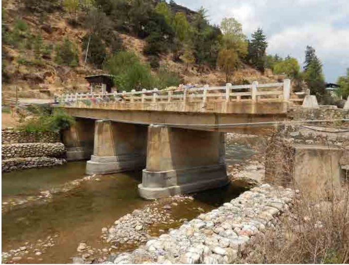
Photo-25 Bridge site survey 2014/4/19 E-1.Dopshari zam Bridge
