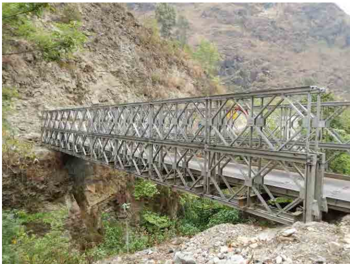
Photo-5 Bridge site survey 2014/4/15~20 A-2.Prakhdrang II Bridge
