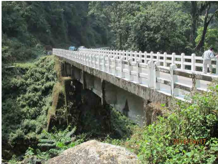
Photo-17 Bridge site survey 2014/4/15~20 B-3.Katley III Bridge
