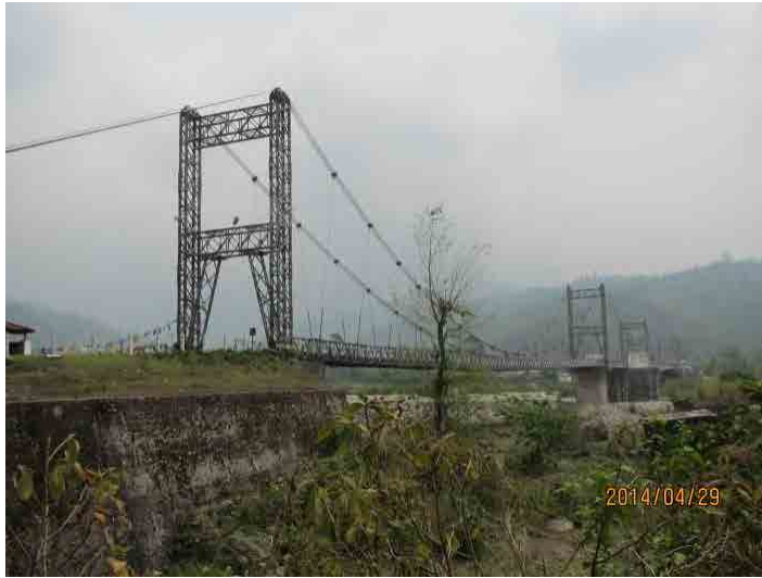
Photo-22 Bridge site survey 2014/4/28~30 C-1.Diana Kuephen zam Bridge
