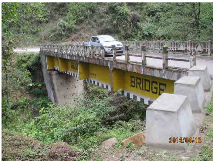
Photo-21 Bridge site survey 2014/4/15~20 B-7.Telegangchu zam Bridge
