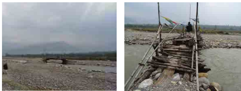
Source: JICA Study Team <Figure7-24>Temporary timber bridge over the Maukhola
