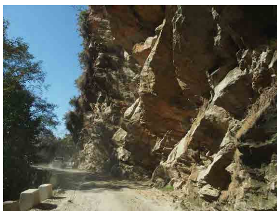
Source: JICA Study Team <Figure5-2> Overhanging rock slope (PNH-1)
