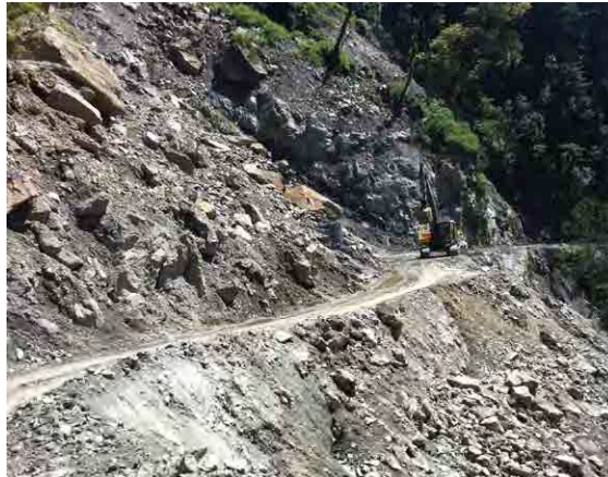
<Figure5-5> States of slope failure points along PNH-4
