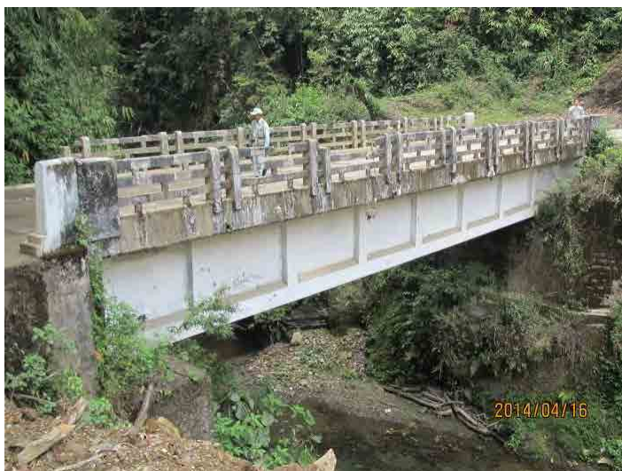
Photo-18 Bridge site survey 2014/4/15~20 B-4.Chaplekhola Bridge
