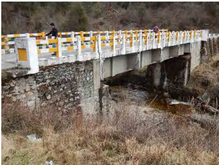
Photo-11 Bridge site survey 2014/4/15~20 A-8.Bong Zam Bridge
