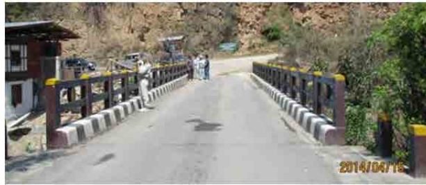
<Figure5-4> Chuzomsa zam Bridge on PNH-1 (Loading capacity=40R)
