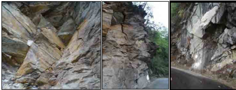
Source: JICA Study Team <Figure6-14>Site condition
