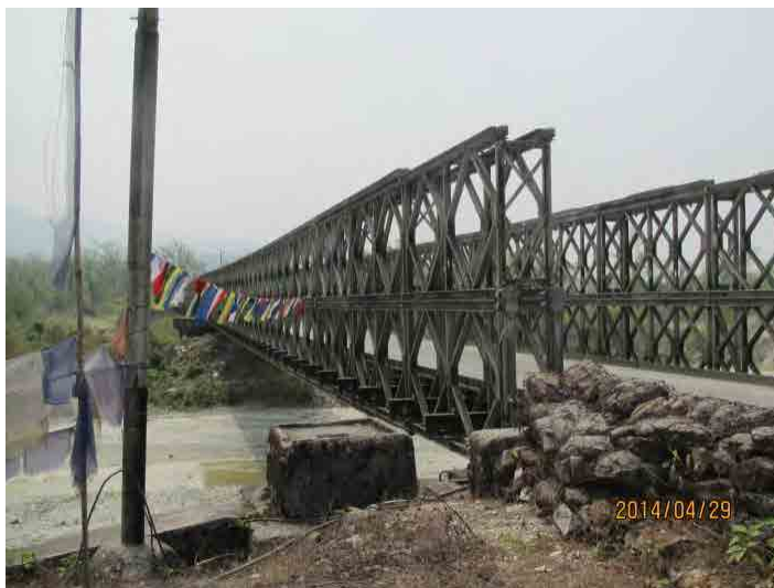
Photo-23 Bridge site survey 2014/4/28~30 C-2.Dramzang zam Bridge
