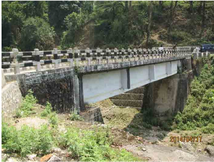
Photo-16 Bridge site survey 2014/4/15~20 B-2.Beteni zam Bridge
