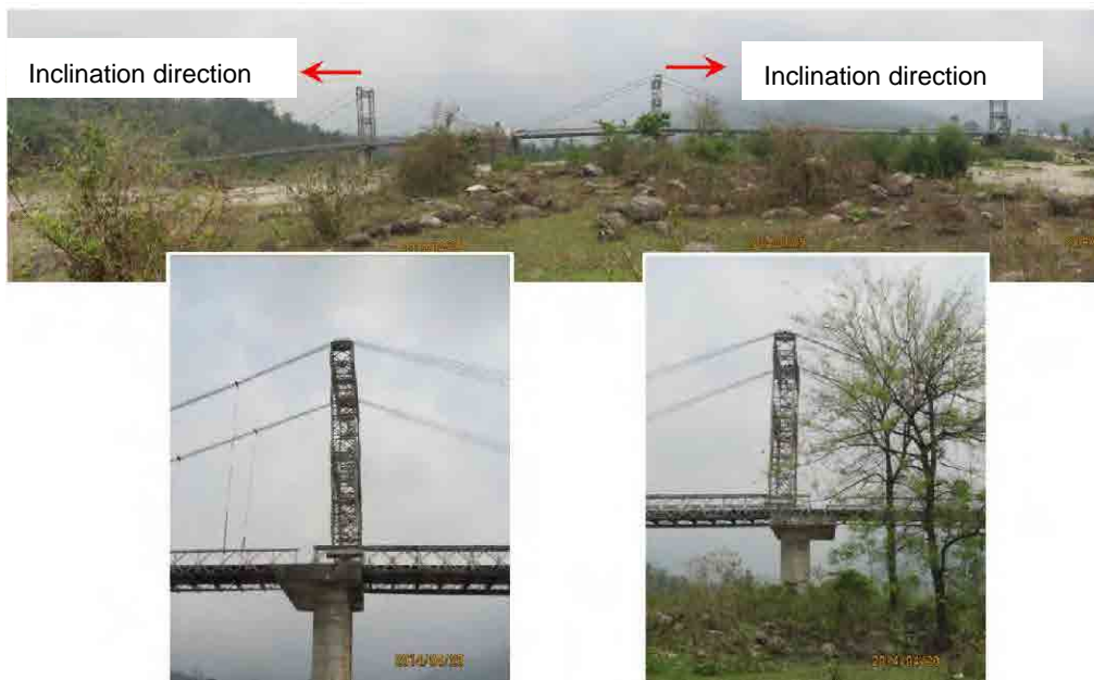
<Figure5-15> States of inclination of the main tower
