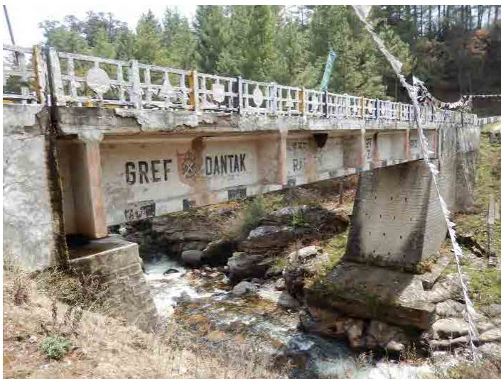
Photo-9 Bridge site survey 2014/4/15~20 A-6.Rabten Zam Bridge
