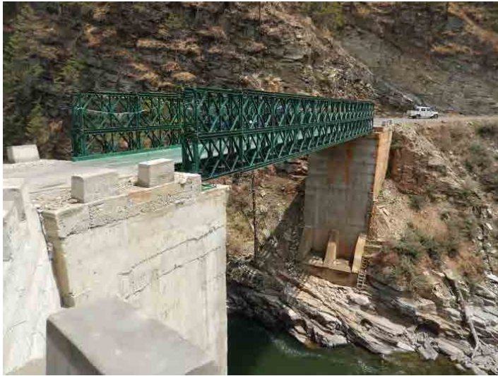
Photo-7 Bridge site survey 2014/4/15~20 A-4.Gektong zam Bridge
