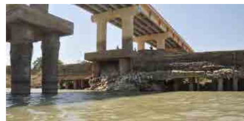
Photo 6.1 Scouring around Cast-in-place Pile Foundation
