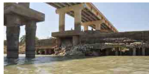
Photo 6.1 Scouring around Cast-in-place Pile Foundation
