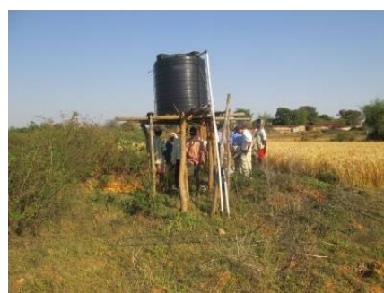
Tank and Wooden Stand
