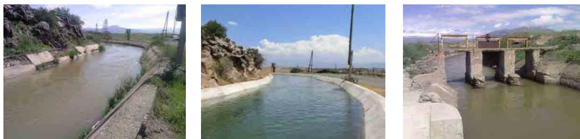
Arzni-Shamiram canal (before rehabilitation)
