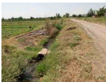
Tertiary canal (earth canal)
