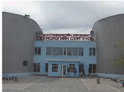
School of Technology Entrance
