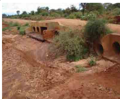
Bridge with pipe culvert installed at the dry up river crossing the road
