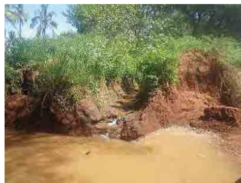
Irrigation canal broken down by flash flood from lateral face
