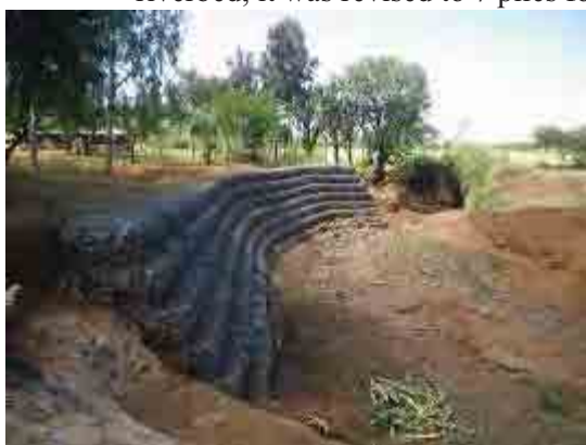
Photo 5.5-1 Revetment by wire mat at the left bank (view from upstream)
