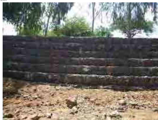
Photo 5.5-2 Revetment by wire mat at the left bank (view from front)
