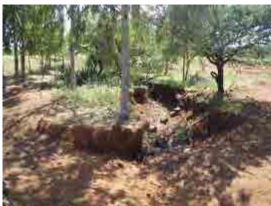
Photo 5.5-7 Hole appeared at the rear side of revetment site
