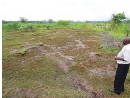
Photo 2.3.2 Broken point of the embankment Canal-C
