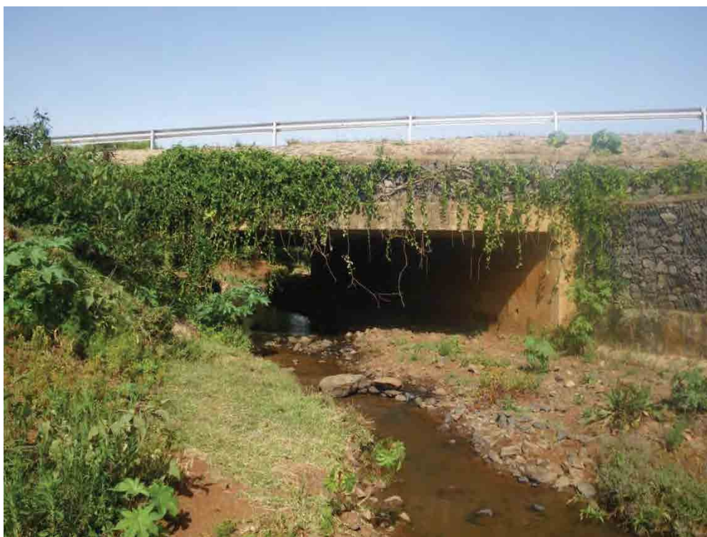
Photo 5.1-3 Culvert Type Bridge
