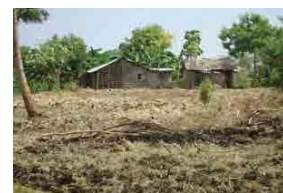
Housing in Marodo Majengo affected by Flooding
