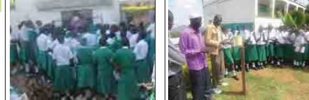
Description : Installation of the rain fall gauge gadget sensor Description : The rain gauge is fitted in its holder at the Itero Girls, the container will be drained after every rainfall in the area.
