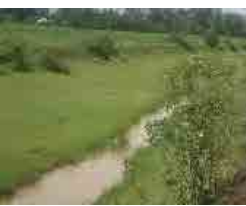
Spillway constructed adjacent to R. Nyando
