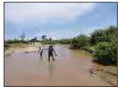
Feeder roads inundated by flood water
