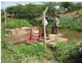
IWASCO water supply intake works
