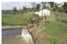
Water supply plant, binged on R. Gucha at Kegati
