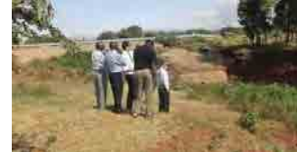
Survey on the eroded river bank at Eastern Maranja River
