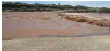
Submerged Gotu Bridge May 10, 2012
