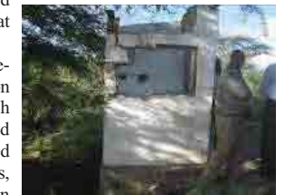
Vandalised Record House
