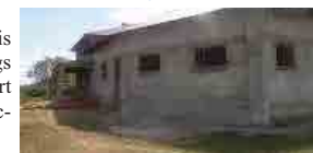
Disaster Centre under construction
