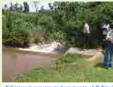
Kibisi weir constructed upstream of R Nzoia
