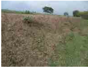
1.5 KM stretch dyke that has been constructed
