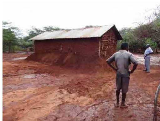
Land elevation after inundation of house Place : Rengesa
