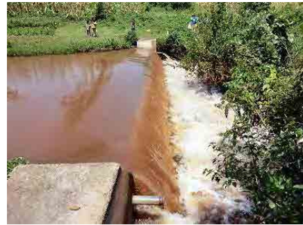
Check Dam (Example of Nzoia River)
