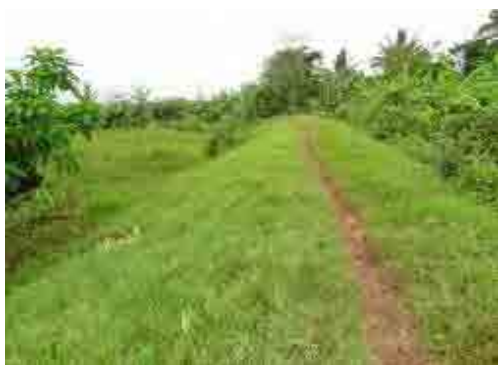
Photo 2.1.1 Embankment of the Canal-C
