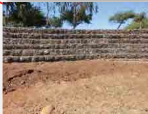
River Bank Protection using Gabion mattress
