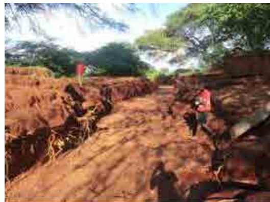
Wash out of land by bank erosion of seasonal river Place: Rekeke
