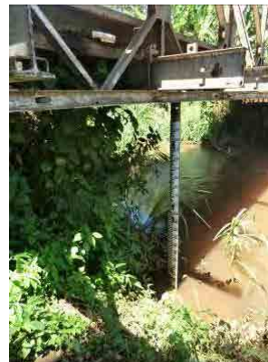
Water Level Gauging Station No. : 3J16 Measure water level of Lumi River. Install device under the pier.
