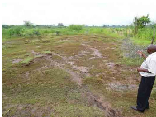
Photo 2.1.2 Broken Point of the Embankment Canal-C
