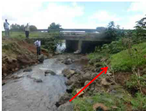
View of upstream from the crossing point of Highway
