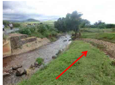
View of downstream from the crossing point of Highway A2
