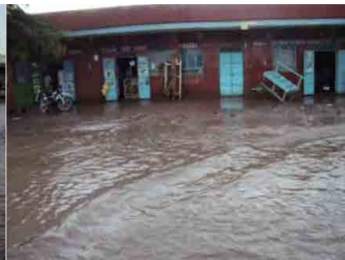
Situation of inundated house
