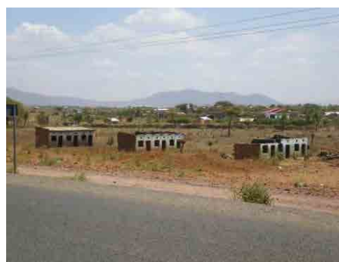
Houses were destroyed by flood
