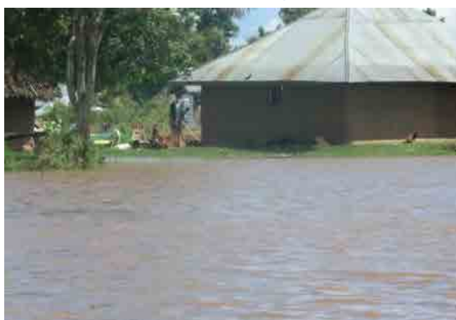
Figure 3.2.5 Flood Characteristics: Damaged riverbank after floods by R. Gucha Migori
