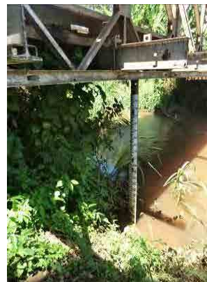
Water Level Gauging Station No.: 3J16 Measure water level of Lumi River. Install device under the pier.
