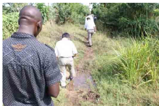
Photo 3.1.4 A point of artificially-destroyed embankment
