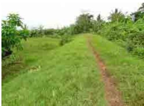
Photo 3.1.1 Embankment of the Canal-C
