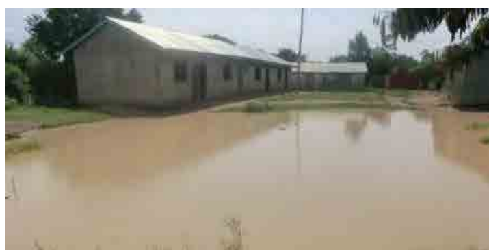
Figure 3.2.8 Flood Characteristics: The rain run-off water flow into the township
