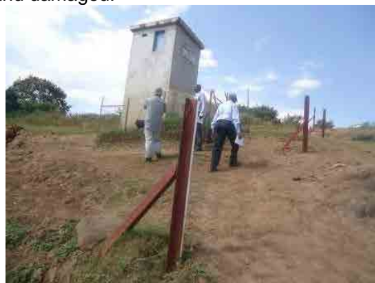
Water Level Gauging Station No.:1KB05 Observation River :Gucha Migori River Special Note : This is an automated gauge station that transmit data to WRMA Regional Office
