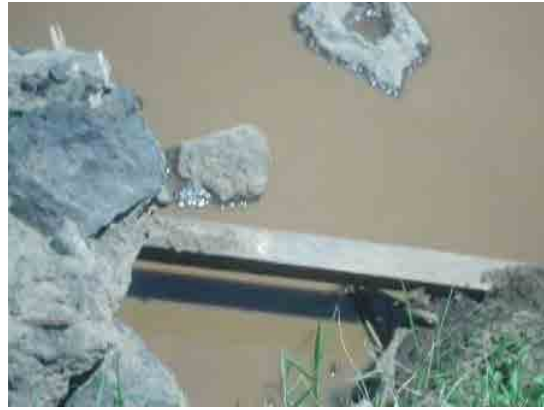
Water Level Gauging Station No.:1KC03 Observation River :Migori River Special Note :Water level gauge is broken off and damaged.
