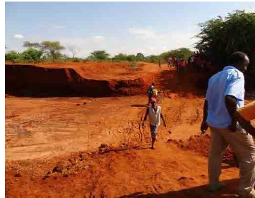
Road Bridge rushed out Place : Rengesa
