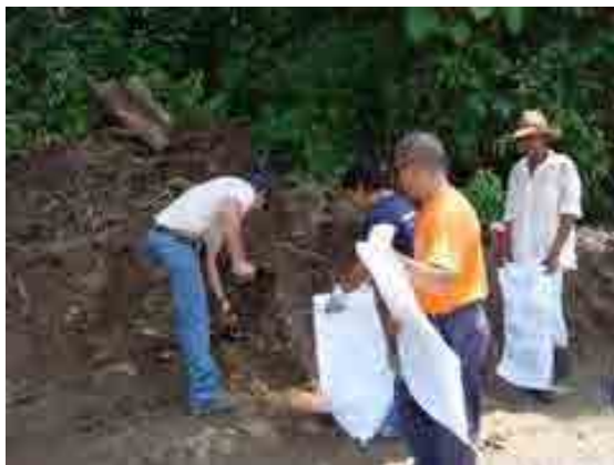
Figure-45 Putting Sand/Soil into Sandbags
