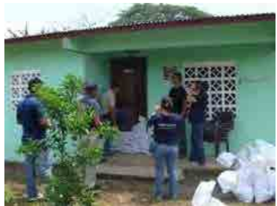
Figure-46 Setting Sandbags in front of Door
