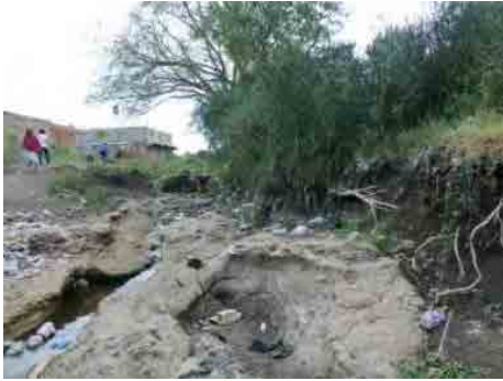
Bank erosion near urban area
