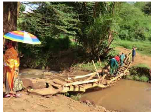
Bridge in the outside of Isiolo Town (Place: Upstream of Isiolo River)
