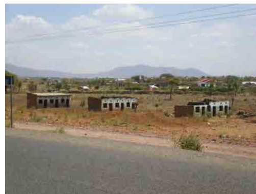
Houses were destroyed by flood
