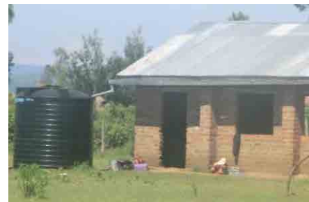
Water tank at Kabuto School, the school is an evacuation place
