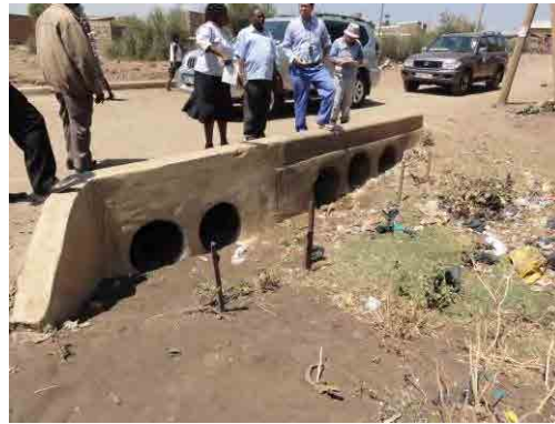
Culvert along the Merire River in Isiolo town
