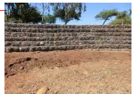
After bank protection using gabion box
