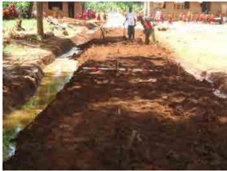
Preparation of the road surface and drainage
