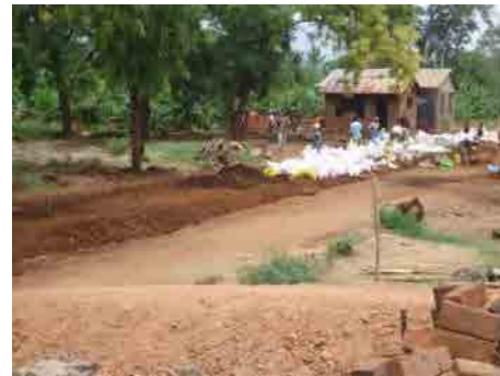
Arrangement of the Do-nou bags on the road
