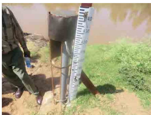
Fig 5 Water Level Gauge Gadget with vandalism proof installed by LOGUMI WRUA
