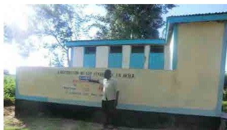
Fig 1 Raised Toilet at Nyora Primary School
