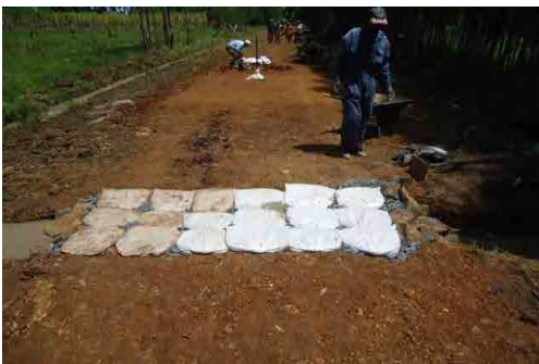
Lay Do-nou bags appropriately and compact
