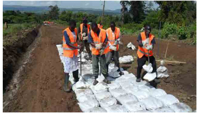
Apply gravel 10 cm thick murrum layer and compact
