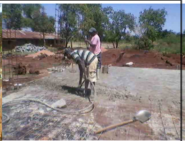
Date: 20-01-2014 Description: Concreting the floor slab
