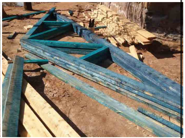
Date: 28-02-2014 Description: Fabrication of roof trusses
