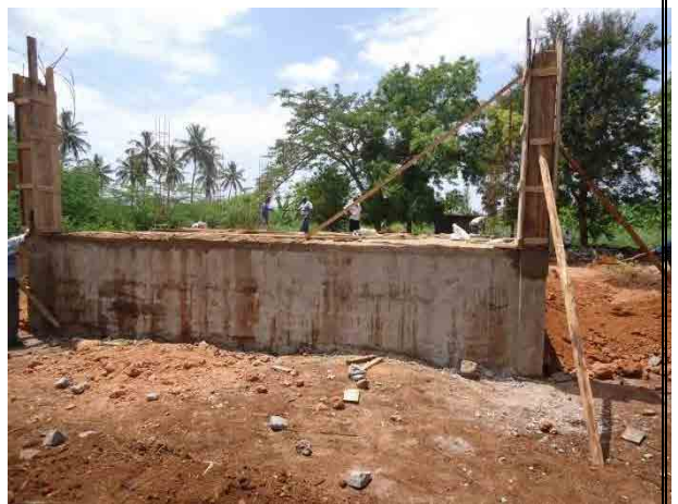
Date: 22-01-2014 Description: Concrete Works for the Columns
