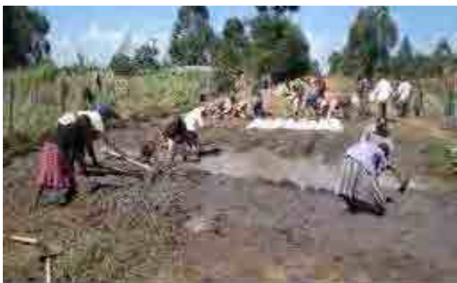
Remove unwanted soft material
