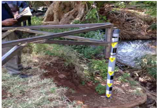
Installation on a metal fabricated stand (Kenya)
