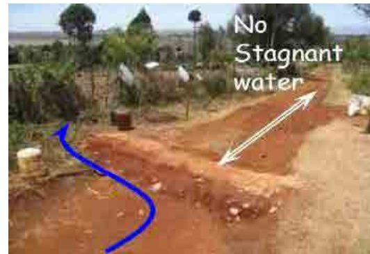
Check that the gradient slopes for water flow
