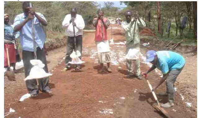
Check camber formation to ensure water is drained away from the carriageway
