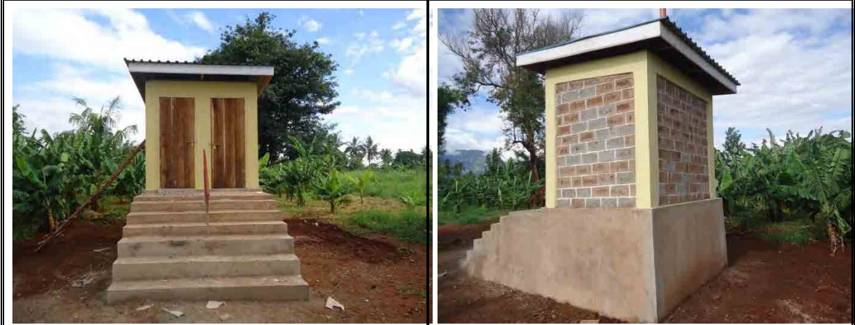
Date :07-04-2014 Description : Finished Toilet front view Date :07-04-2014 Description : Finished Toilet side view
