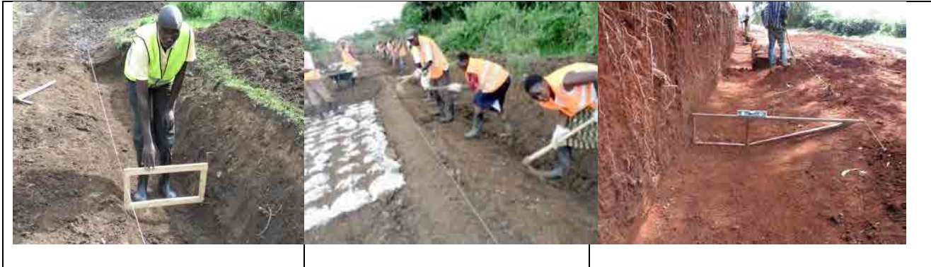
Control ditch excavation width using ‘ditch template’
