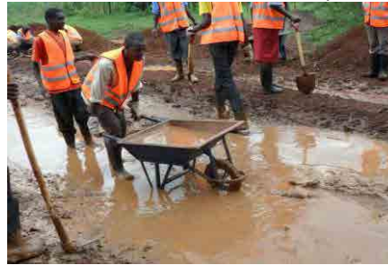
If there is mud, remove and dispose off
