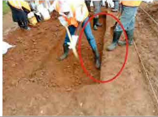
Lay Do-nou bags appropriately and compact
