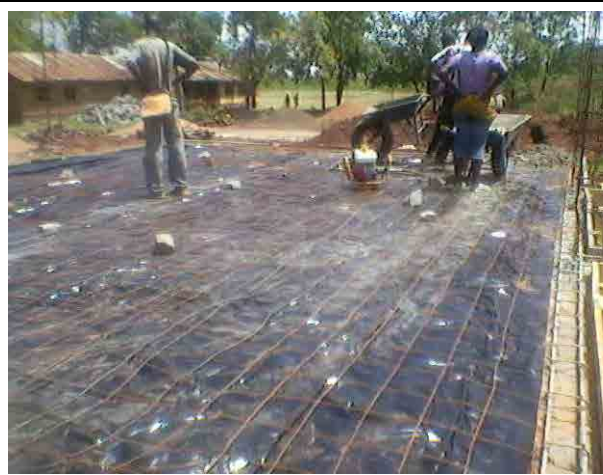
Date: 20-01-2014 Description: Preparation for foundation the floor slab, BRC 142 and DPC Polyethylene sheeting
