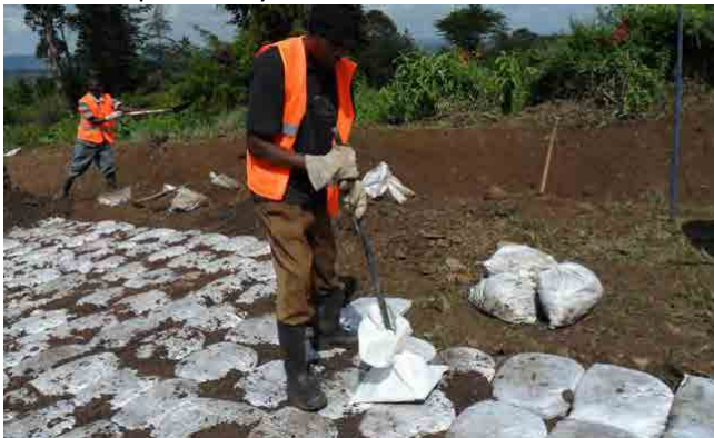
If the soil is too dry, water it to facilitate compaction
