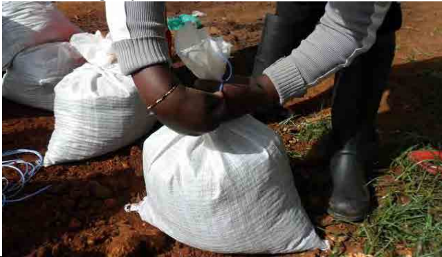
Fill the spaces between the Do-nou bags and compact the fill independently
