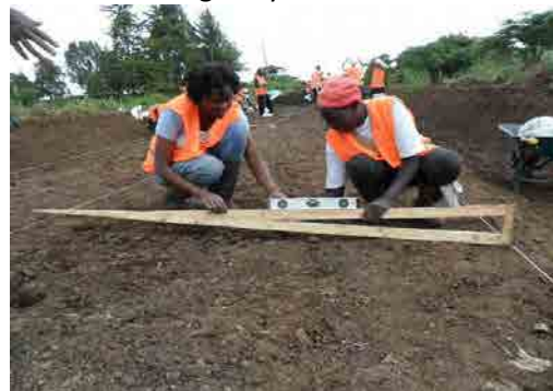
Check camber formation to ensure water is drained away from the carriageway
