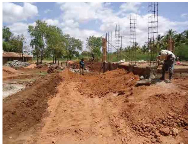
Date: 22-01-2014 Description: Reinforcement for the Columns
