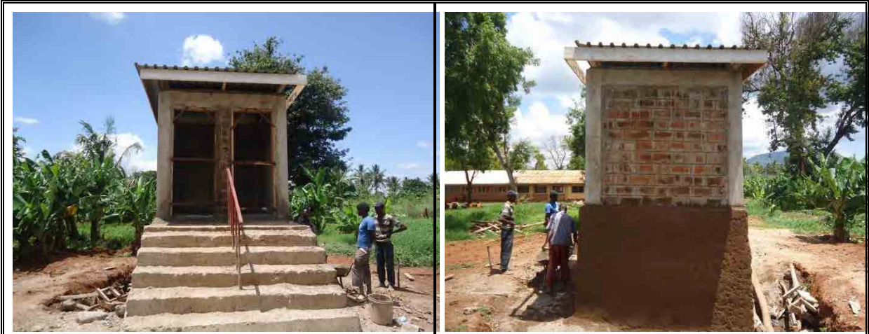
Date :18-03-2014 Description : Preparation for door installations Date :18-03-2014 Description : Finishing Works
