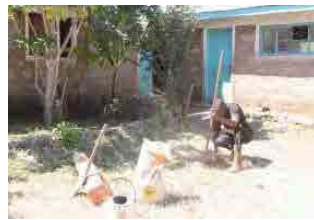
WRUA member digs the ground for pillar.
