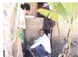
Mr. Jared connects wire and pipe
