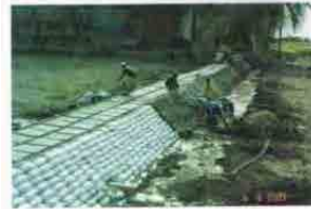
Construction of the embankment in dry season (Height : 1.5 m, 7,500 Do-nou used)
