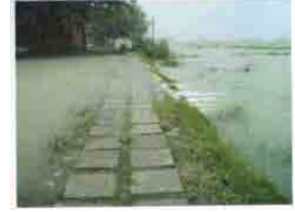
The embankment during rainy season (It was stable.)
