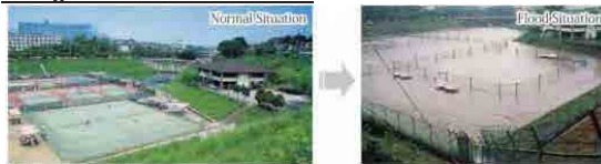
Rainwater storage and infiltration facility
