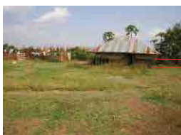
The wall of house was soaked by flooded water and collapsed. Depth of flood water
