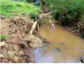
Water Level Gauging Station No.:5DA04 Observation River: Eastern Marania River Special Note: Water level gauge is broken off and damaged.
