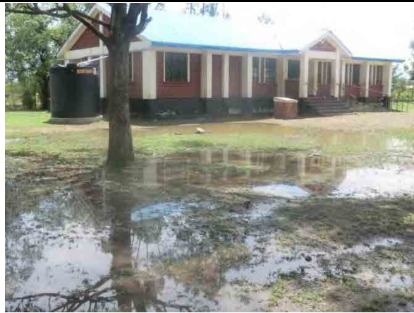
Description : Raised Evacuation centre above flood depth
