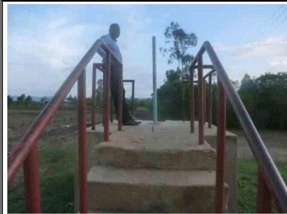
Description: Borehole at Kojiem village hand pump was removed and kept at the chair's house for fear of vandalism after the bolt that holds the hand-pump to the slab was breached
