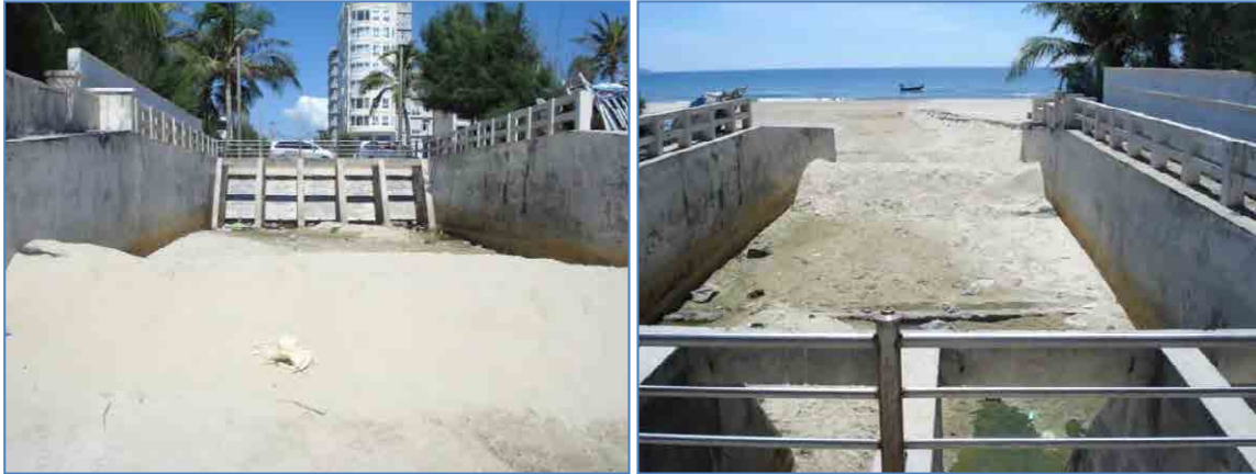
Figure 2.3 Combined Sewer Outfall CX01
