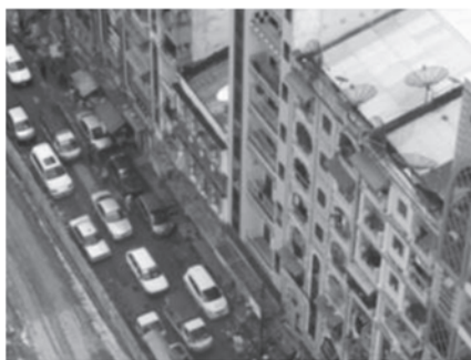
Figure 6.2.3.7 Parallel parking on narrow roads in the CBD
