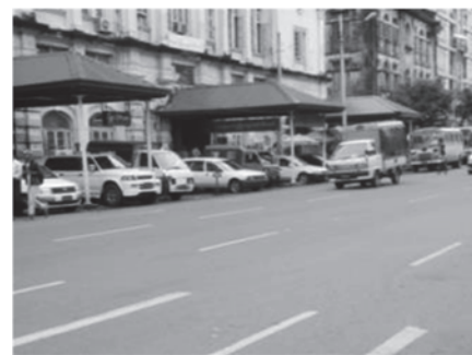
Figure 6.2.3.8 Back-in style parking on the high-standard trunk road in the CBD
