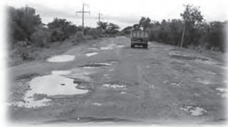
Road No.7 (Hlegu TS)
