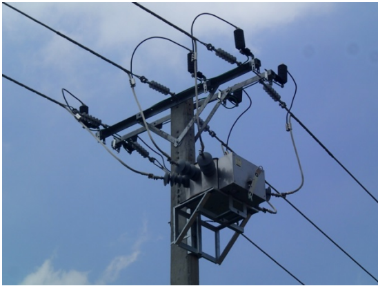
Fig. 8.4-8 Pole Mounted Type Switch
