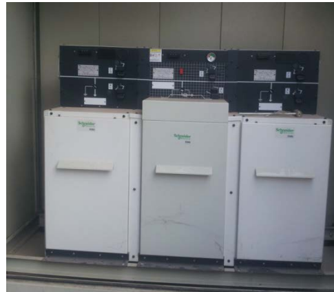
Fig. 8.4-9 Indoor Type Switch
