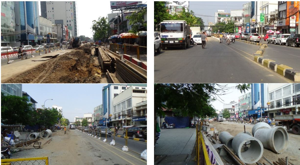
Fig. 4.2-1 Ongoing Construction Work of Underground Sewage Pipe
