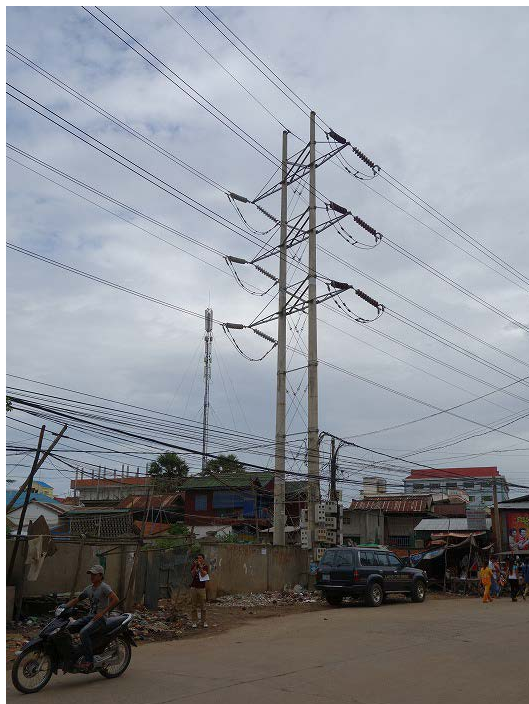
Fig. 4.1-5 Concrete Pole near Toul Kork S/S
