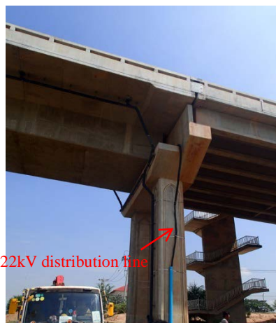
Fig. 4.4-4 Existing Cable laid on the Bridge
