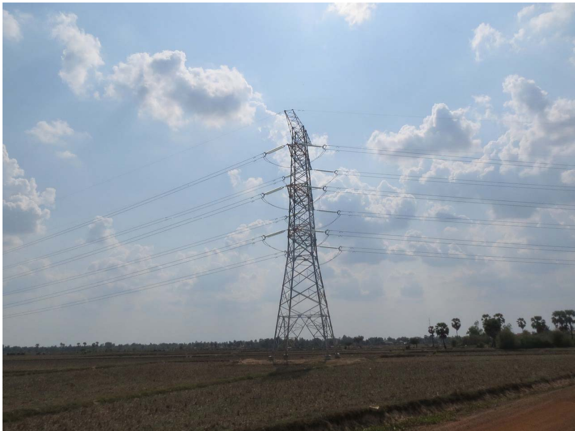
Fig. 8.1-3 230kV Steel Tower in the Midpoint of NPP and WPP
