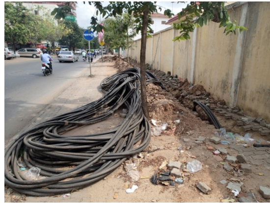
Fig. 8.4-4 Underground Line (under construction)
