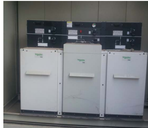
Fig. 8.4-9 Indoor Type Switch
