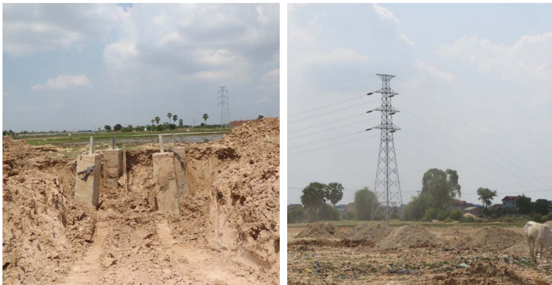
① [115kV TL construction is stopping]
