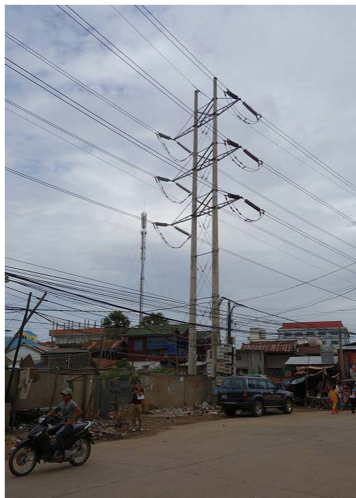
Fig. 7.1-38 Field Survey Route Photograph of 115kV_Route3
