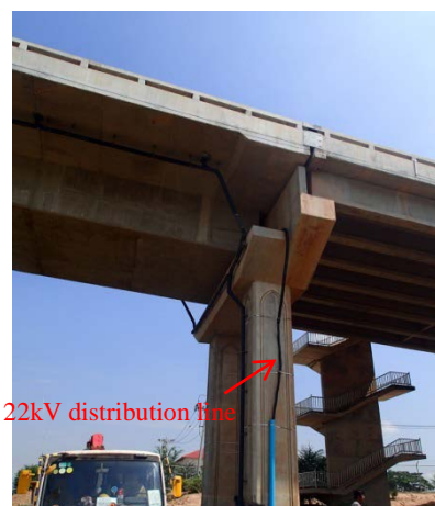
Fig. 4.4-4 Existing Cable laid on the Bridge
