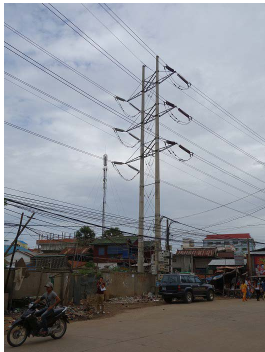
Fig. 4.1-5 Concrete Pole near Toul Kork S/S
