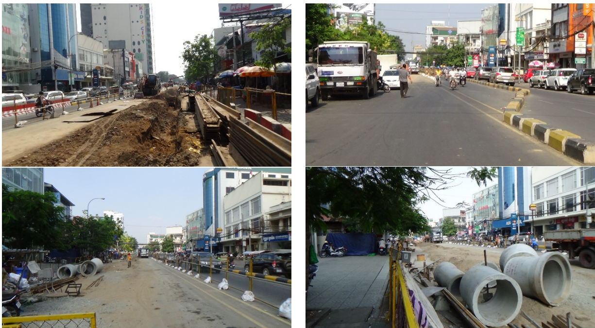
Fig. 4.2-1 Ongoing Construction Work of Underground Sewage Pipe
