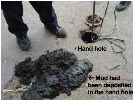
Pict-3.2.2 The inside of the hand hole that has not been maintained [3-8]
