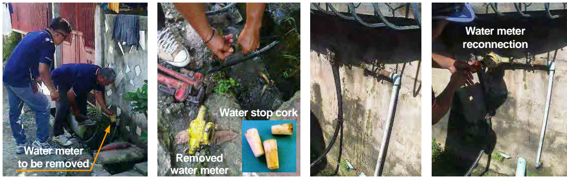
Pict-2.2.3 Disconnection work (Left 2 pictures) / Reconnection work (Right 2 pictures) [2-47]
