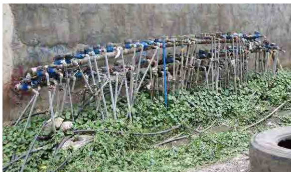
Pict-2.2.1 Example of Stub-Out installation: 82 water meters on one Stub-Out
