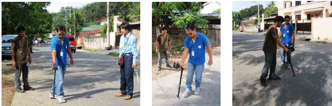
Pict-3.5.3 Water leakage survey by D305
