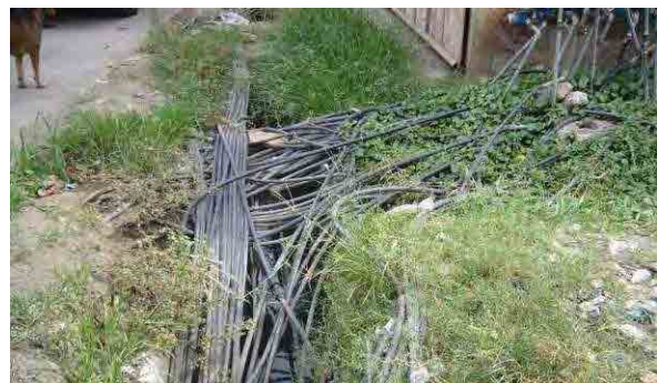
Pict-2.2.1 Example of Stub-Out installation: 82 water meters on one Stub-Out
