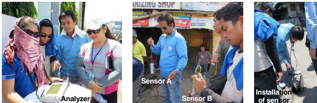
Pict-3.5.1 Water leakage survey by AQUASCAN 610 [3-45]
