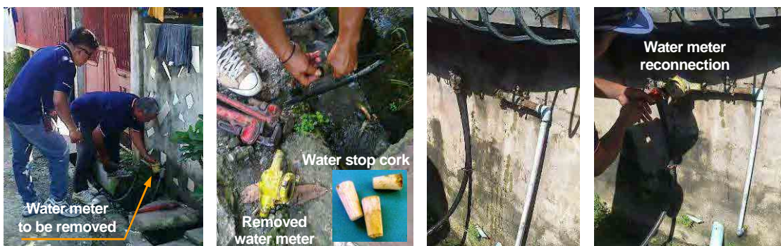
Pict-2.2.3 Disconnection work (Left 2 pictures) / Reconnection work (Right 2 pictures)
