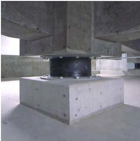
Fig.5.Seismic isolators
