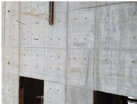
EXPOSED CONCRETE FINISH : 良好な仕上げ
