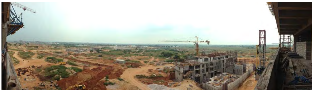
CAMPUS OVERVIEW FROM CHEMICAL BUILDING
