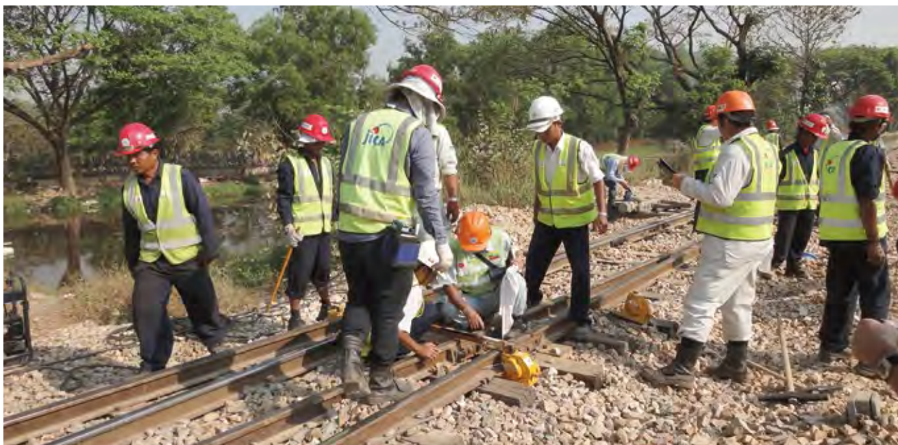
Myanmar: training on gauge measurement, part of the Project on Improvement of Railroad Service and Safety of Railway.
