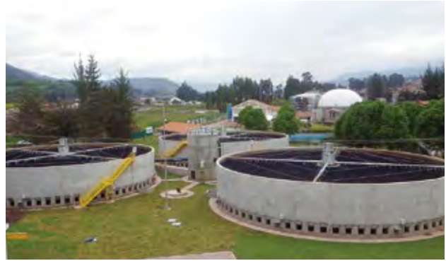
Sewage Plant in Cusco funded by ODA Loan (Peru)
