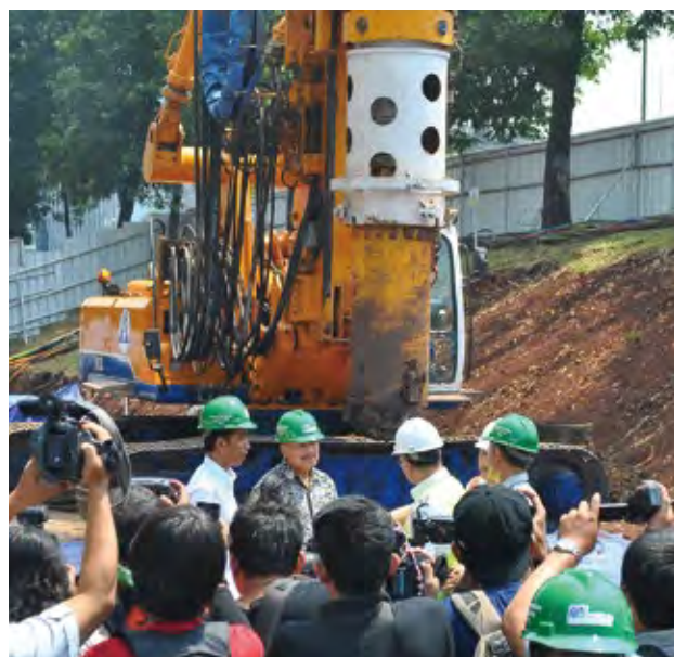
Groundbreaking ceremony for the North-South line (ODA Loan) of the Jakarta Mass Rapid Transit (MRT), which is expected to help relieve the capital's traffic jams.
