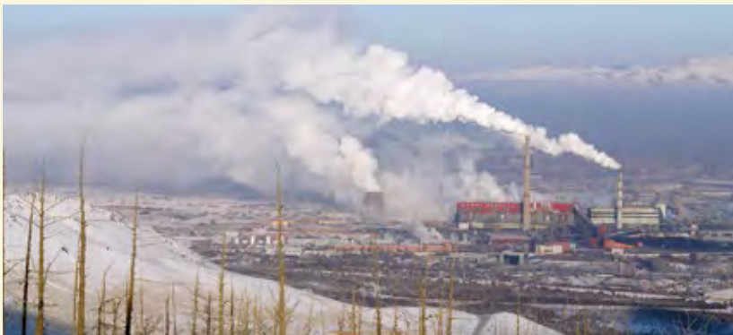
One of the major sources of air pollution: emission from a combined heat and power plant
