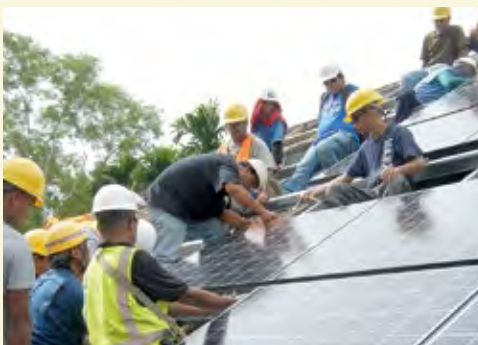
Installation of solar panels in Micronesia
