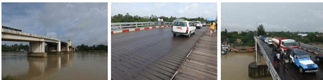
Existing Thaketa Bridge
