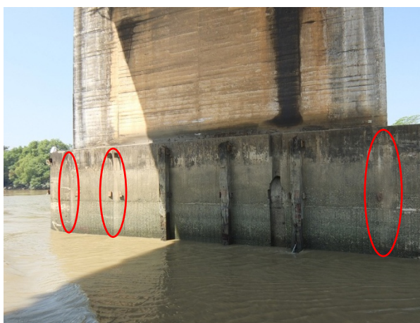
Figure 2.3.10 Collapse of Fenders on the Pier of the Existing Thaketa Bridge
