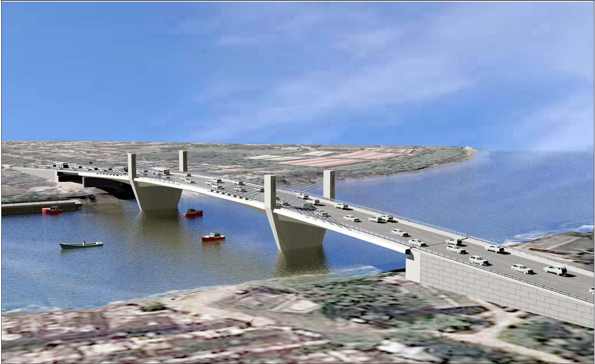
New Thaketa Bridge (PC Extradosed Bridge) Perspective
