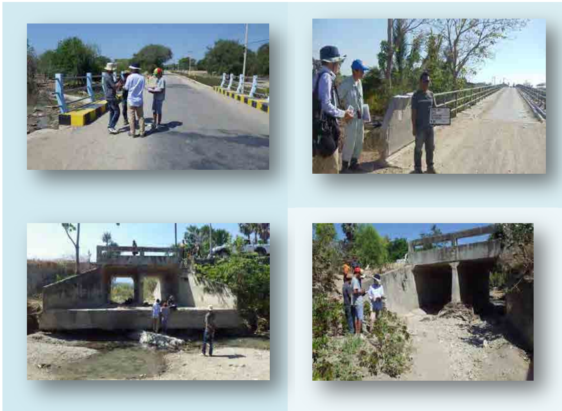
Figure 3.10.2 Picture of Bridge Resister Database Site Survey
