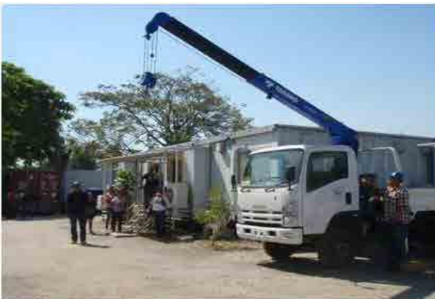
Demonstration of Truck with Crane at Outside
