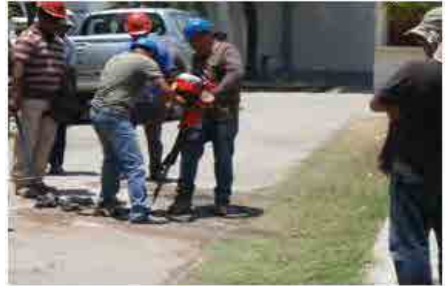
Actual Repairing Training for Pot hall on the Road (Sep. 2014)
