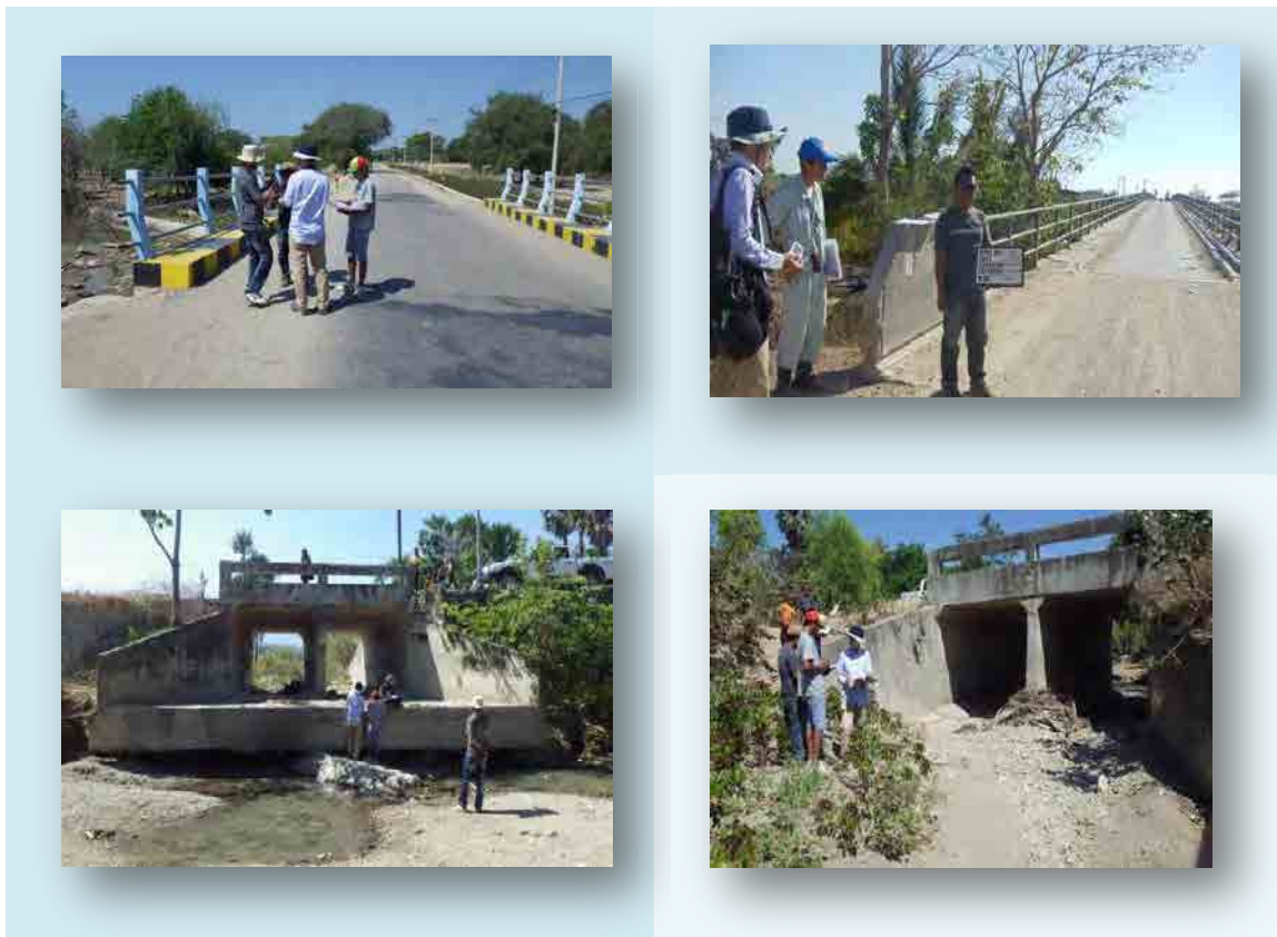
Figure 3.10.2 Picture of Bridge Resister Database Site Survey
