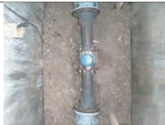
Installation of electromagnetic flow meter
