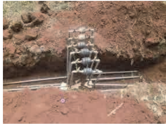
Service pipe setting
