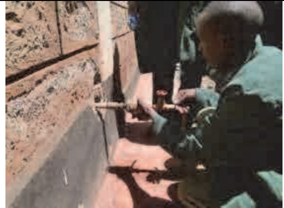
Replacement of customer meter
