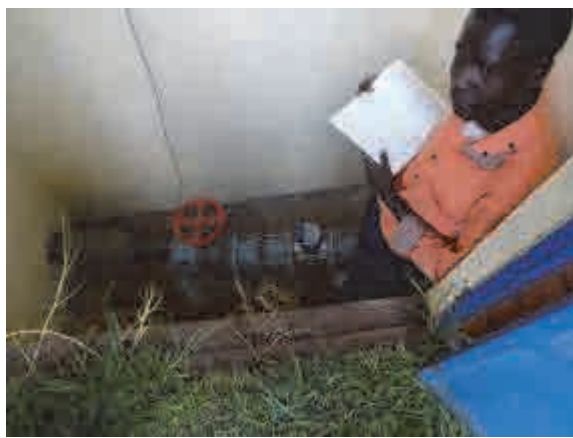
Measuring flow volume at electromagnetic flow meter
