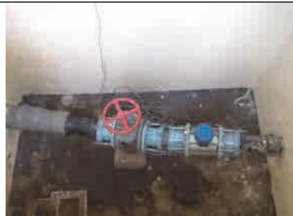
Installation of electromagnetic flow meter
