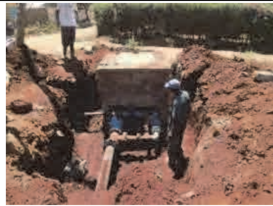
Construction of measuring chamber
