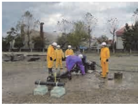
OJT of distribution pipe connecting
