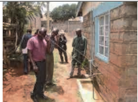
OJT of leak detection with listening stick
