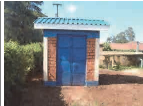
Construction of measuring hut
