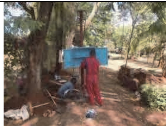
Installation of telemetric monitoring system
