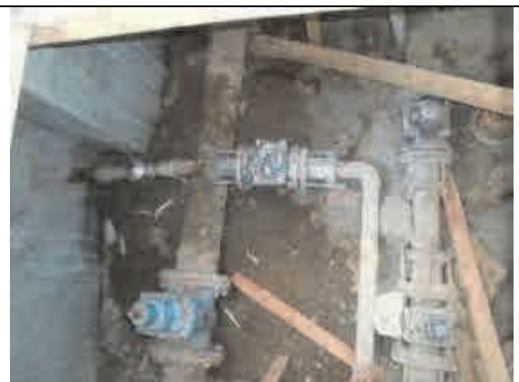
Installation of pressure reducing valve
