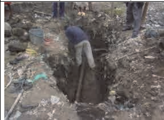
Repair leakage from distribution pipe
